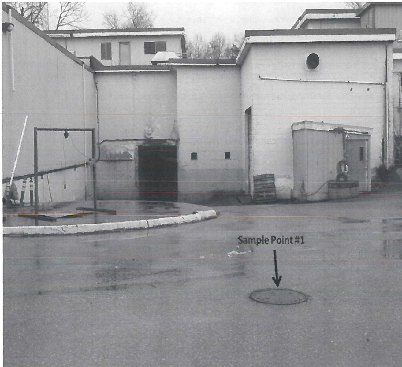
Photograph of Sample Point 1:
