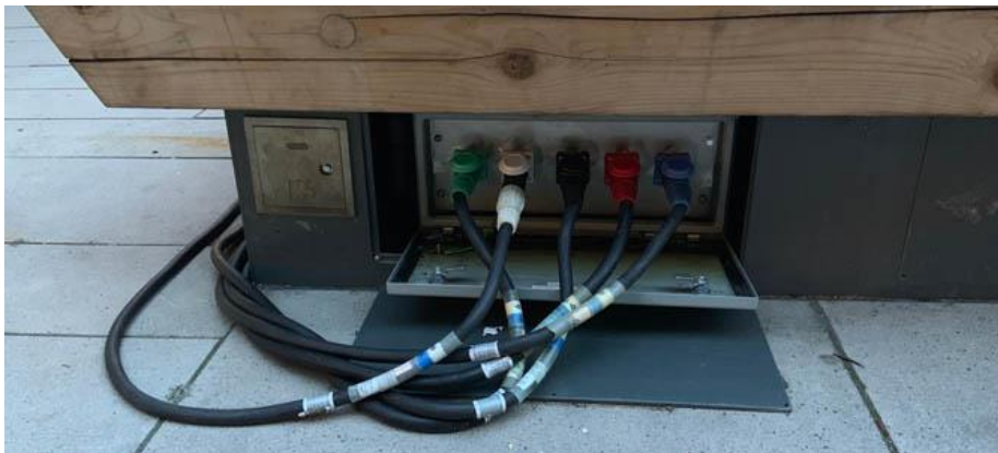
Film power kiosk at the Vancouver Art Gallery. Credit: City of Vancouver
