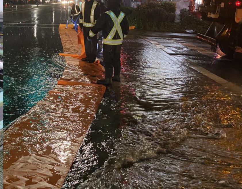
WWTP Emergency Storage / Langley SSO
