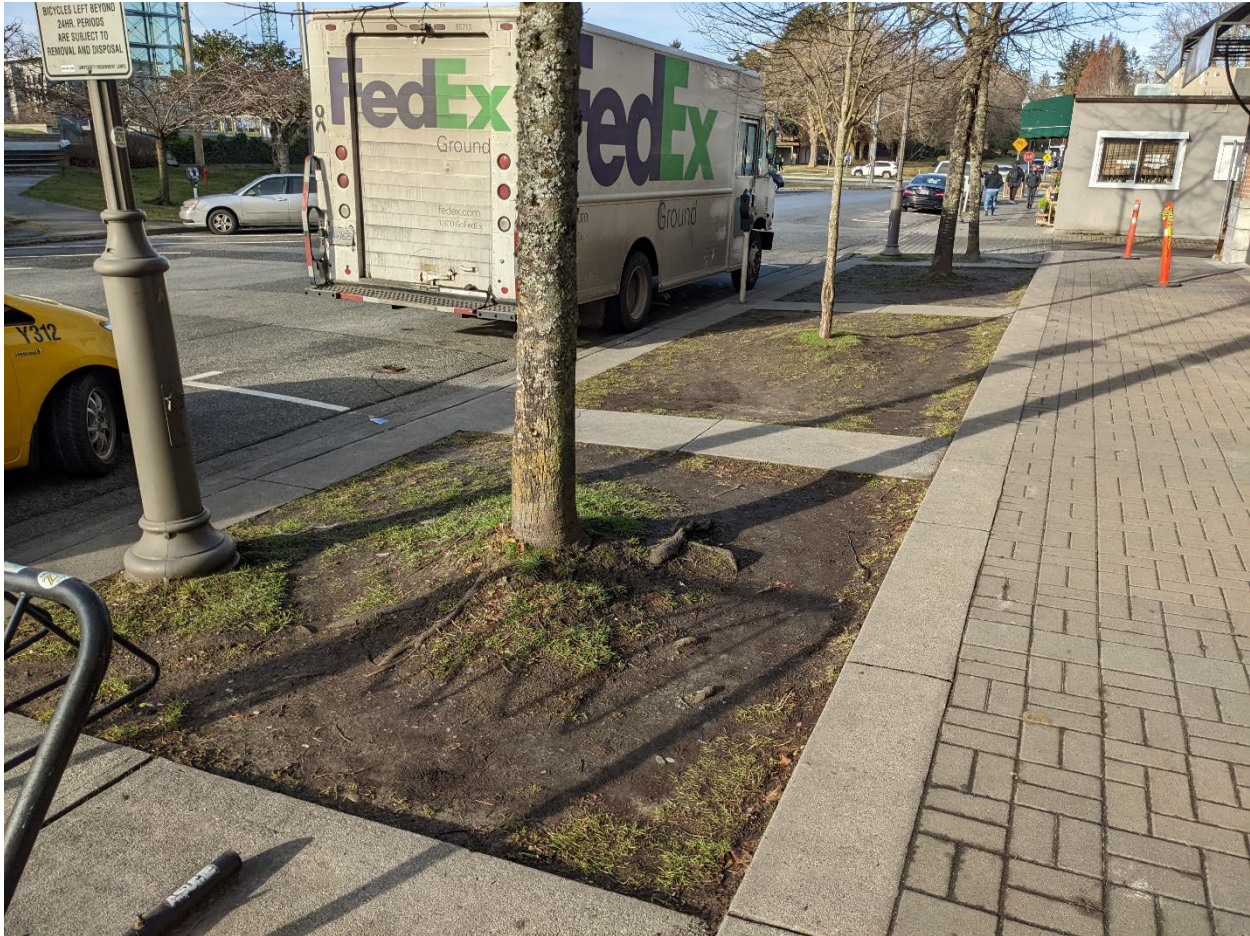
Mudpits looking North on Eastern side of Western Parkway
