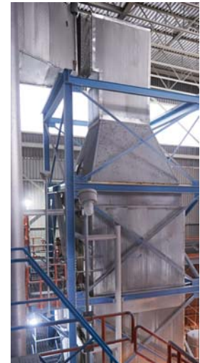
Economizer Replacement Project
