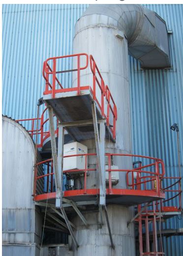
Stack Sampling Ports
