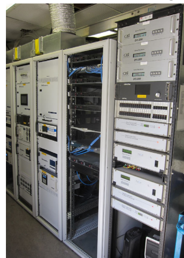
Continuous Emission Monitoring Analyzers
