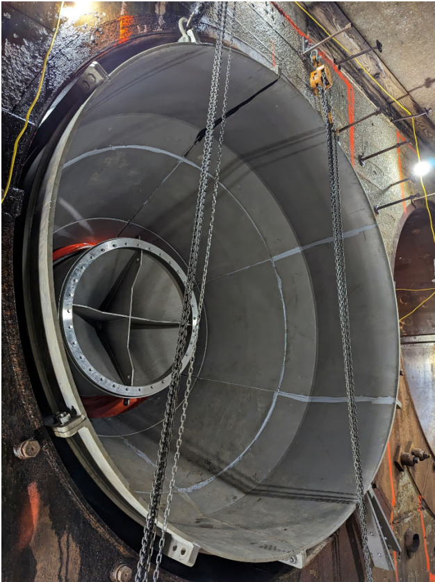
West Lower Outlet Fixed Cone Valve Hood
