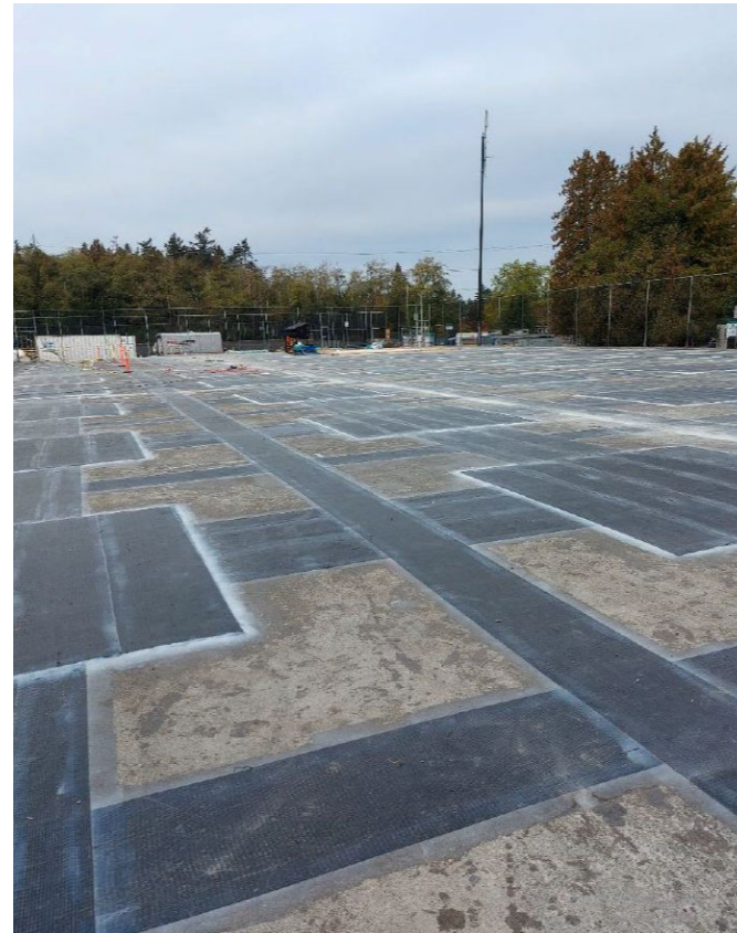
Application of the fiber reinforced polymer strengthening system on the rooftop
