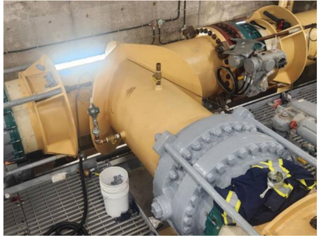
Oxifree Application at 14th Avenue Crossover Chamber
