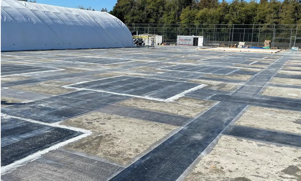
Pebble Hill Reservoir FRP Roof Strengthening – September 2022
