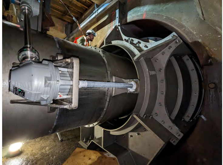
West Lower Outlet Fixed Cone Valve Hood
