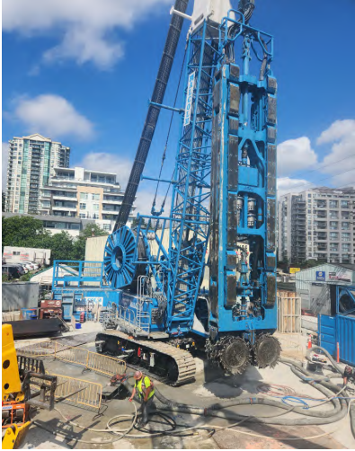
Hydromill working on a slurry wall panel at the North shaft
