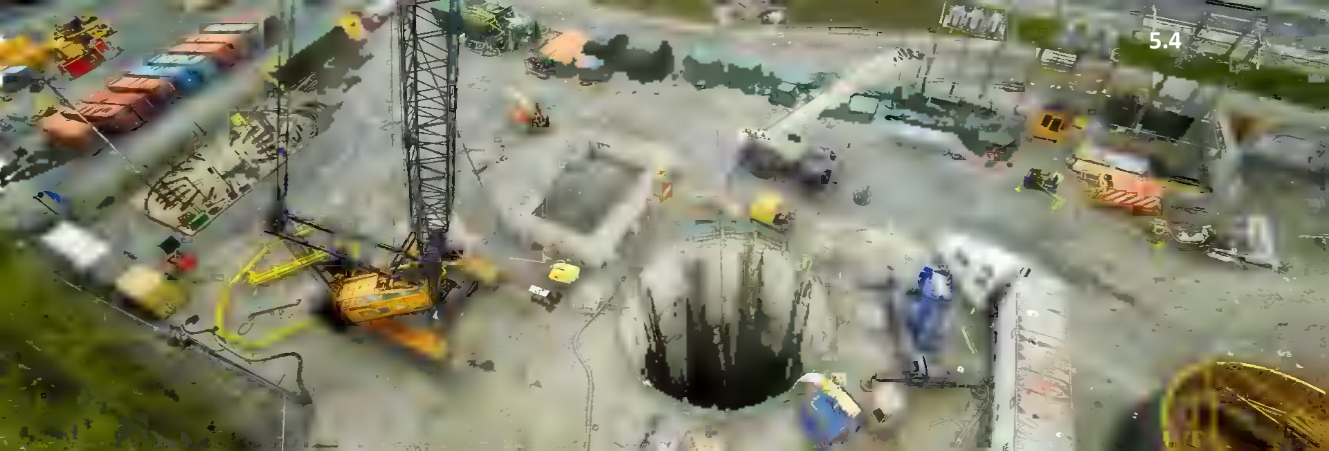
Port Mann Water Supply Tunnel Shaft
