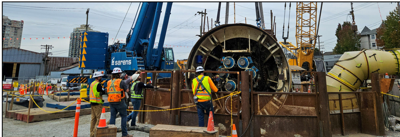
Annacis Water Supply Tunnel Boring Machine
