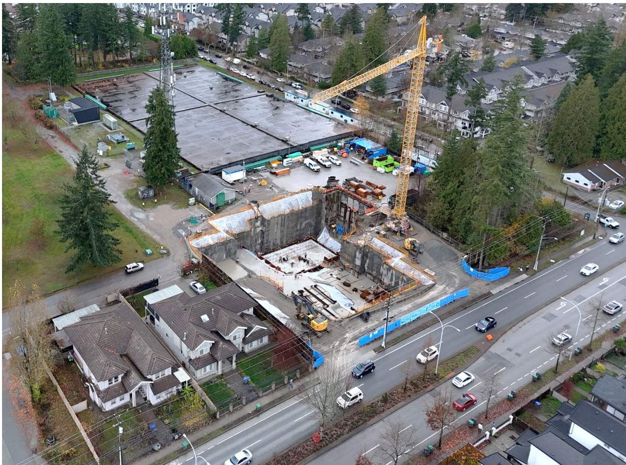
Excavation for the Newton Pump Station Replacement, November 2025
