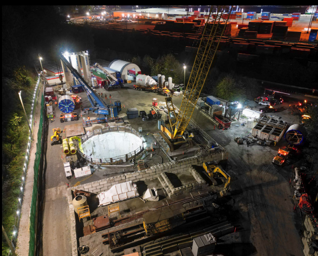
Annacis Water Supply Tunnel South Shaft
