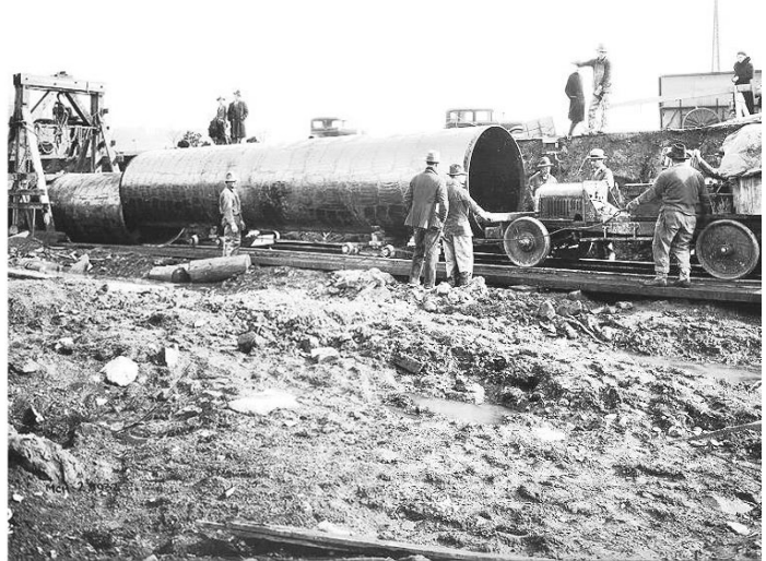
Installation of original water main in Stanley Park, 1932
