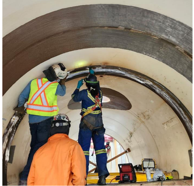
Robson to Guildford Section – 3.2 m diameter steel pipe weld inspection
