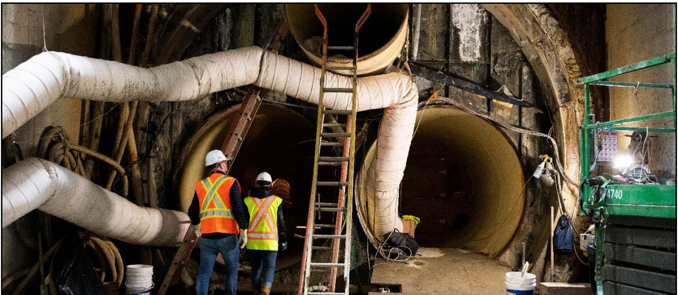
Second Narrows Water Supply Tunnel
