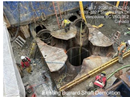
Existing Burrard Shaft Demolition
