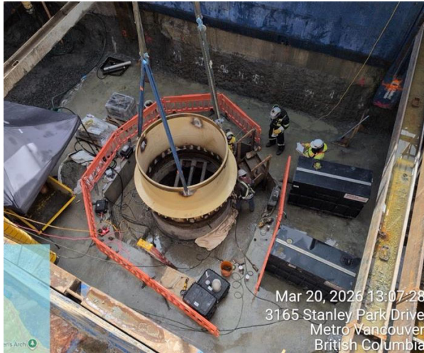
Work currently underway
