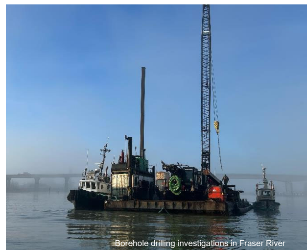
Borehole drilling investigations in Fraser River
