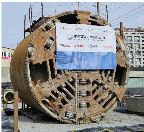
Tunnel Boring Machine
