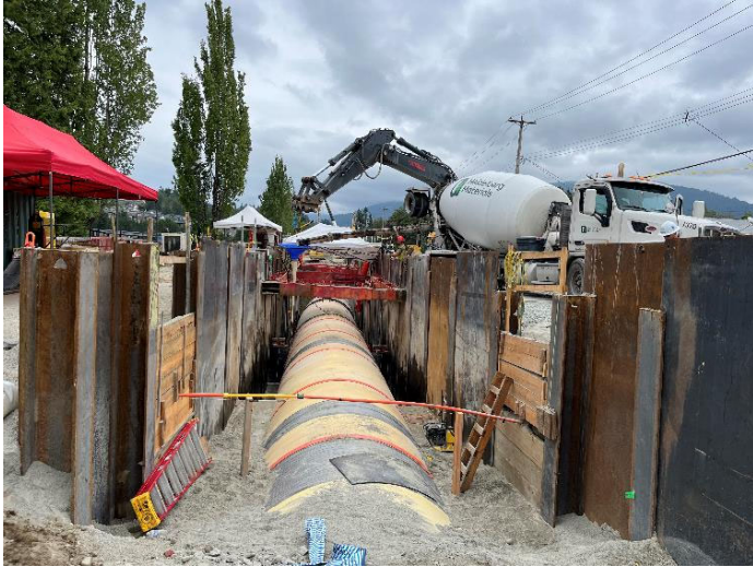
Robson to Guildford Section – 3.2 m diameter steel pipe installation
