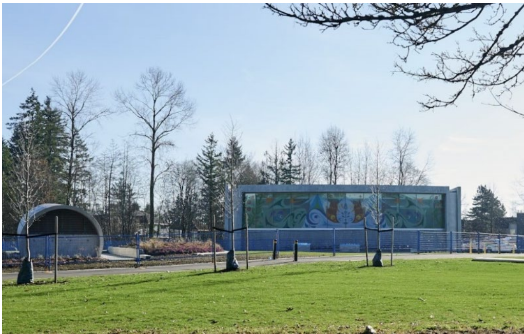
Photo 4 – Maintenance Building with Mural and Egress Structure
