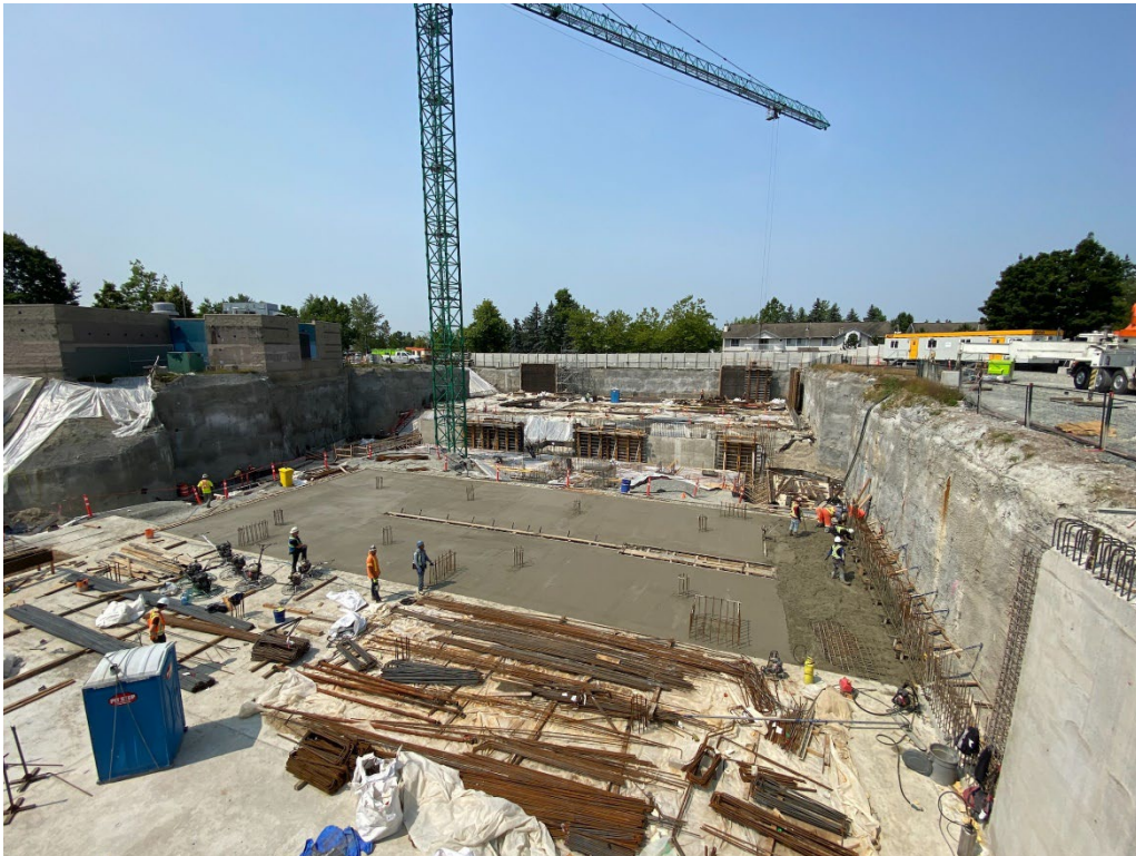
Photo 1 – Construction of Reservoir Cells Adjacent to Surrey Pump Station
