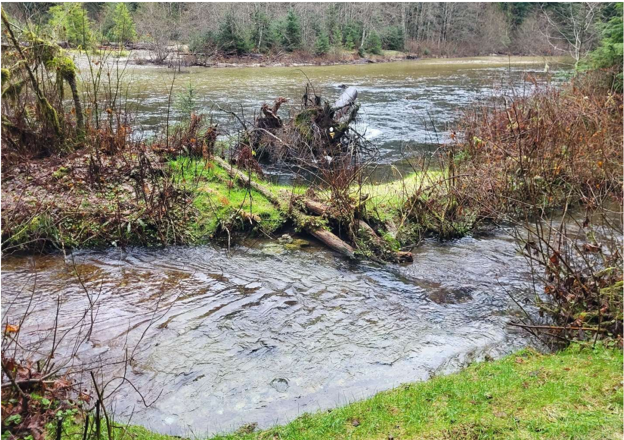
FIGURE 2 JUNIOR CREEK OUTLET CHANNEL AT SITE OF REPAIR WORKS
