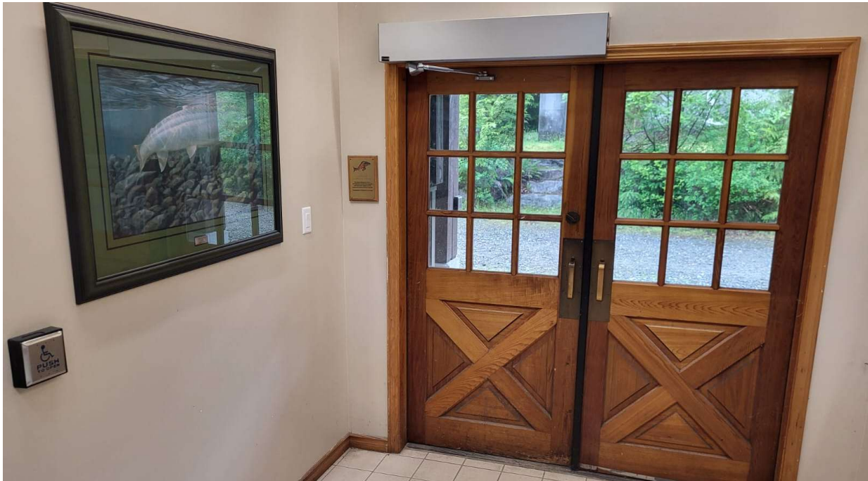
FIGURE 19 COMPLETED FOYER ENTRANCE WITH AUTOMATIC OPENING DOORS
