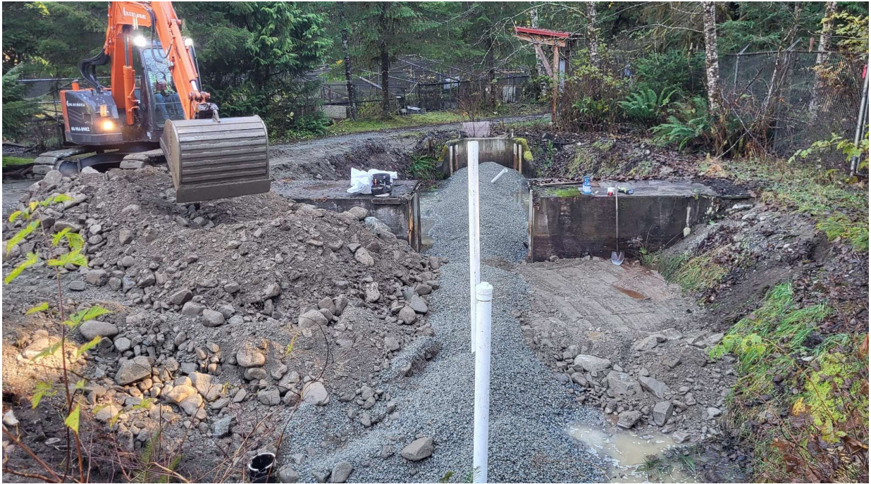
FIGURE 21 GROUND WORKS AND PLUMBING INSTALLATION AT THE HATCHERY
