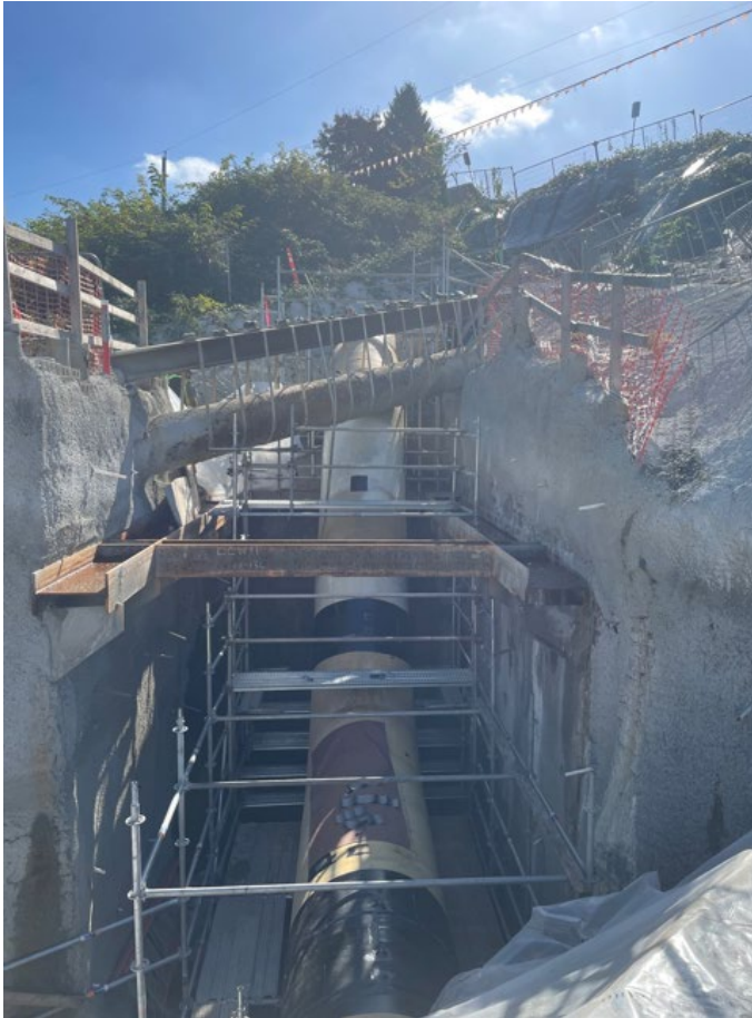
Figure 1 – Tie-in of Capilano Main No.7 - South Side of Burrard Inlet in the City of Burnaby
