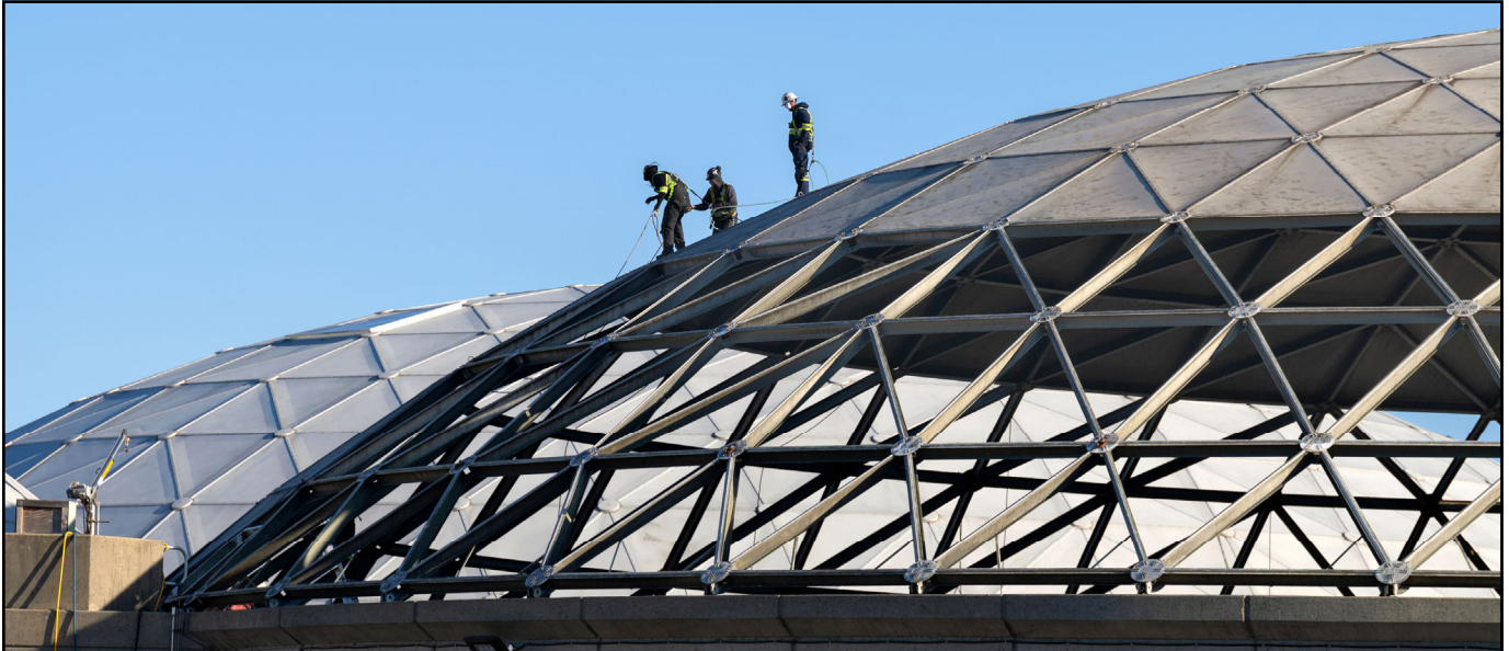
A crew works on the installation of the new trickling filter domes at Annasis Island Wastewater Treatment Plant
