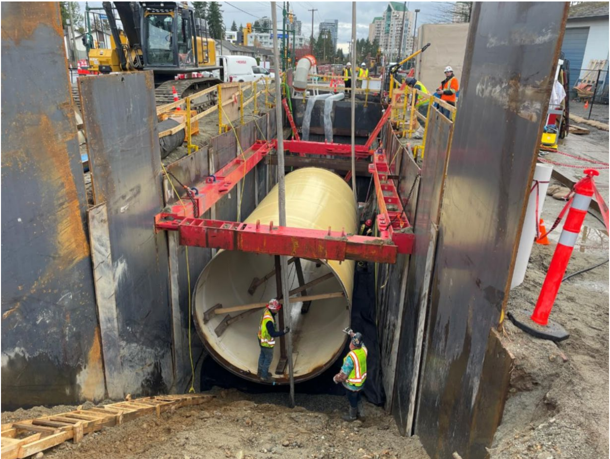
Figure 2. Coquitlam Water Main – Robson to Guildford pipe installation.
