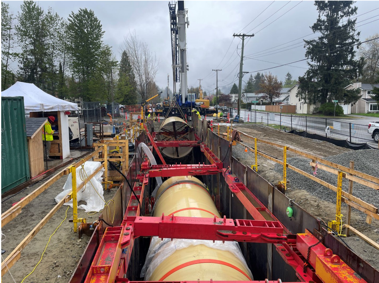
Figure 1. Coquitlam Water Main – Robson to Guildford Section pipe installation
