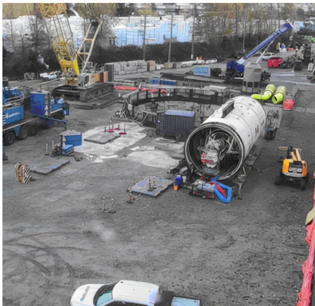
Figure 15: Annacis Water Supply Tunnel - Tunnel boring machine
