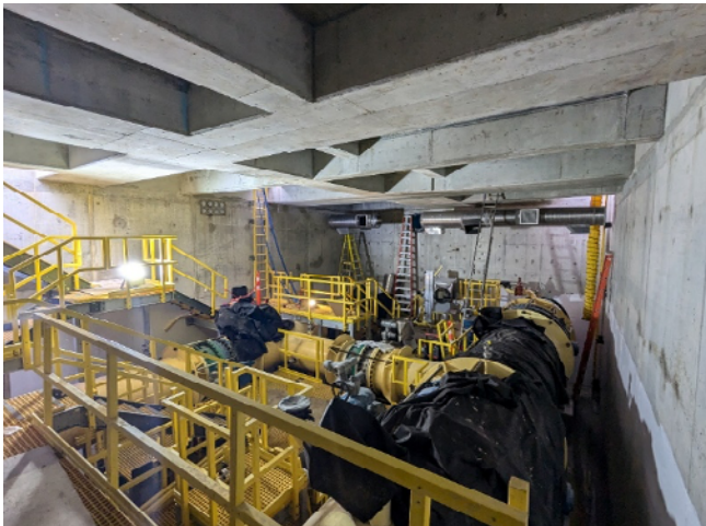
Figure 18: Kennedy Newton Water Main – Installation of Piping and Valves within the Large Underground Valve Chamber
