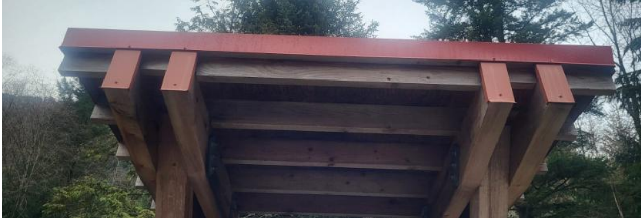
FIGURE 23 ROOF FLASHINGS FOR THE INFORMATION SIGNAGE
