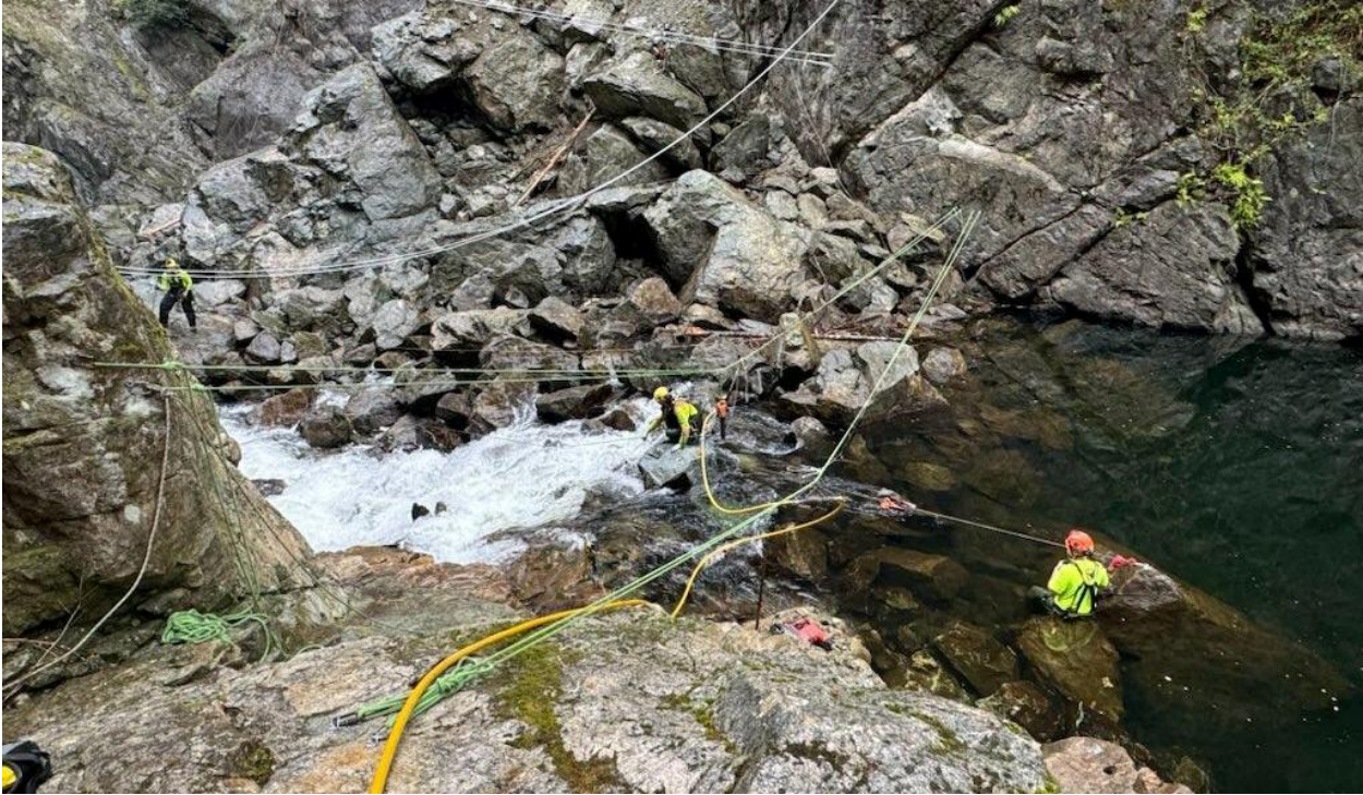
FIGURE 1 SEYMOUR ROCKSLIDE MITIGATION WORKS DURING SUMMER LOW FLOWS 2024
