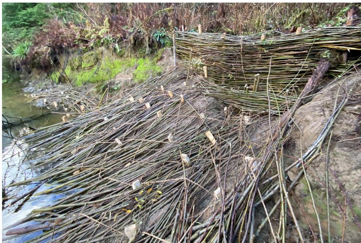
FIGURE 5 JUNIOR CREEK OUTLET COMPLETED WILLOW SPILING BANK PROTECTION STRUCTURE
