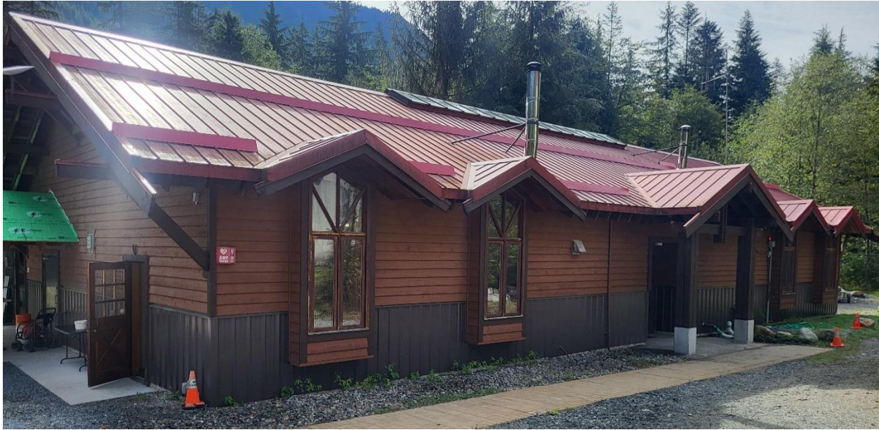
FIGURE 20 COMPLETED WATERPROOF SIDING ON THE HATCHERY BUILDING
