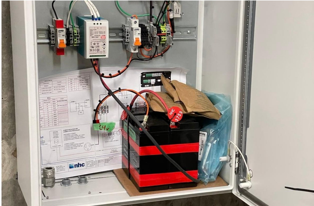
FIGURE 26 FLOW METER INSTALLED IN THE AERATION TOWER PIPE ROOM
