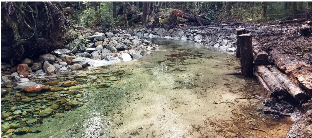
FIGURE 3 JUNIOR CREEK INLET FOLLOWING COMPLETION OF REPAIR WORKS
