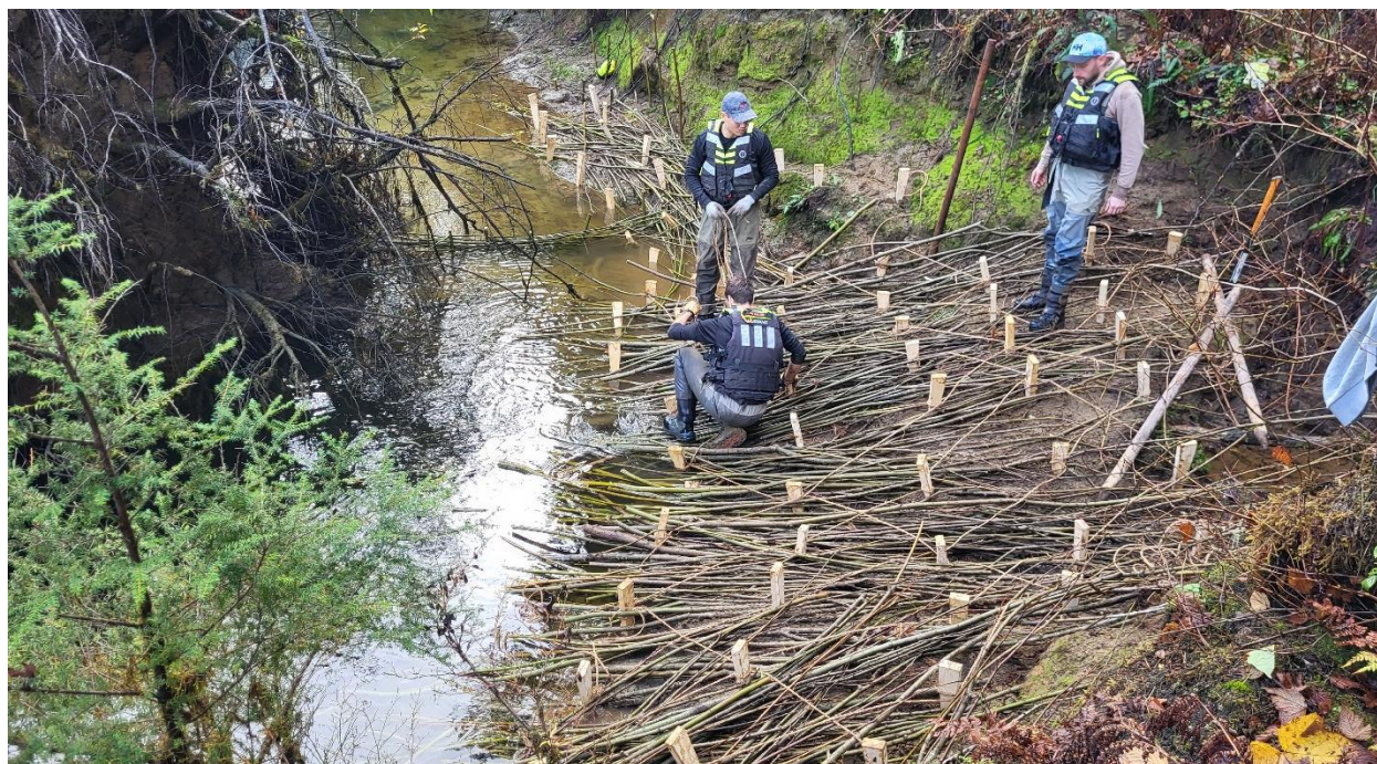
FIGURE 4 JUNIOR CREEK OUTLET DURING INSTALLATION OF WILLOW SPILING
