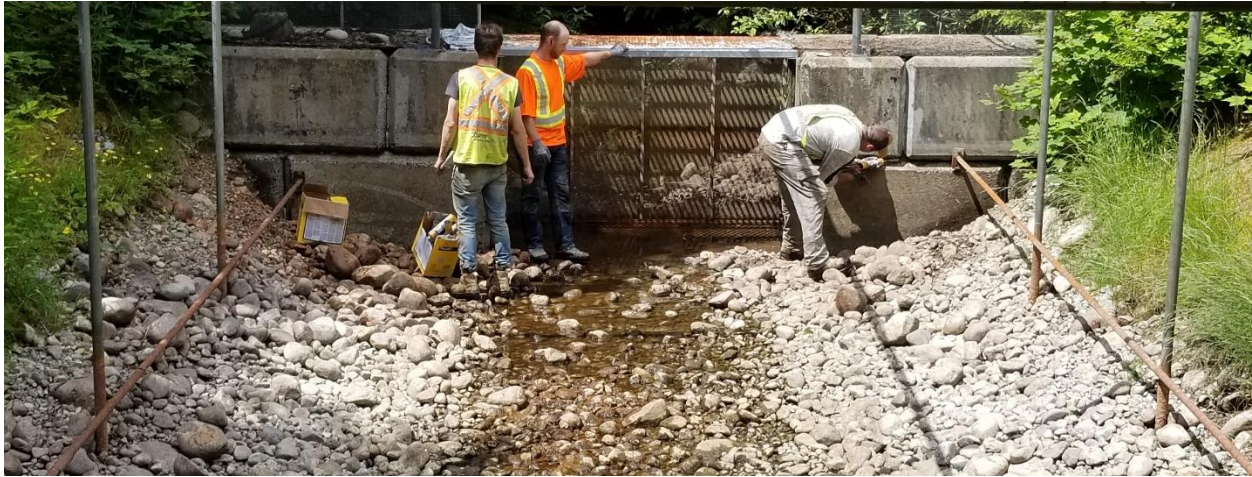
FIGURE 19 CONTRACTORS UNDERTAKING WEIR AND HEADWALL REPAIRS
