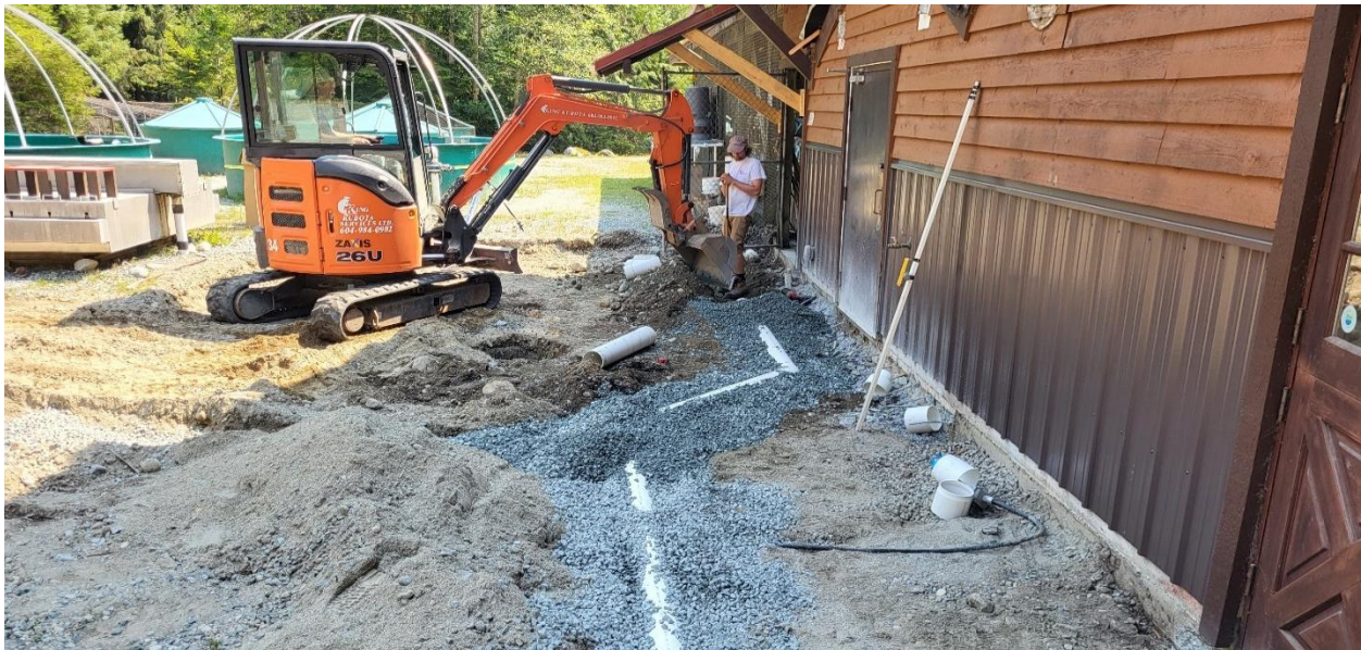
FIGURE 21 PERIMETER DRAINAGE WORKS AROUND HATCHERY BUILDING
