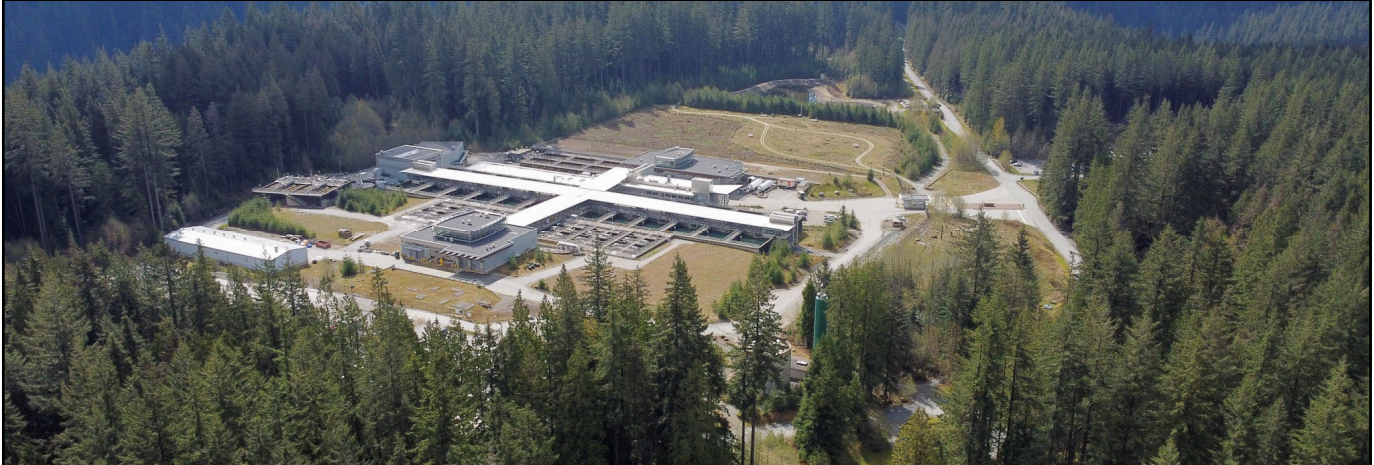
Seymour Capilano Filtration Plant
