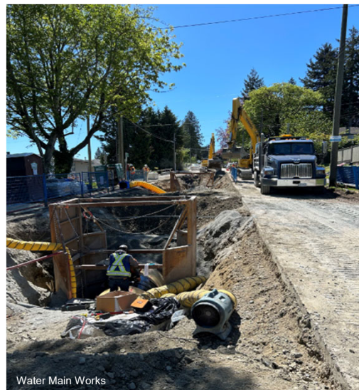
Water Main Works
