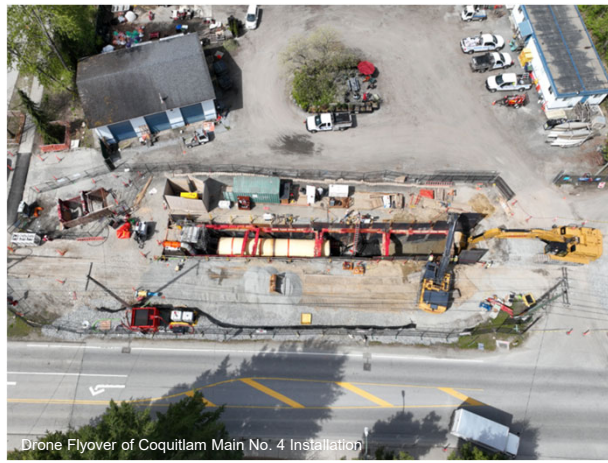
Drone Flyover of Coquitlam Main No. 4 Installation
