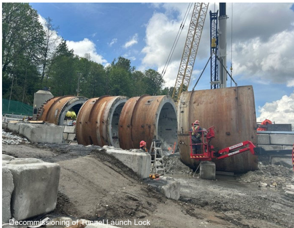
Decommissioning of Tunnel Launch Lock
