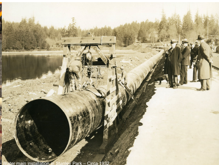
Water main installation in Stanley Park – Circa 1932
