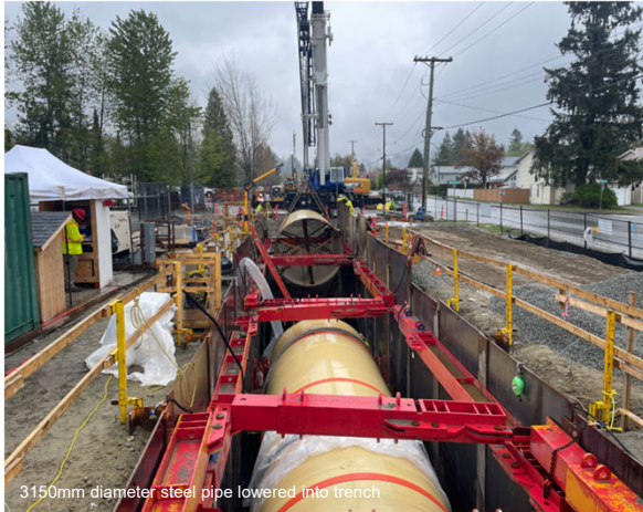
3150mm diameter steel pipe lowered into trench
