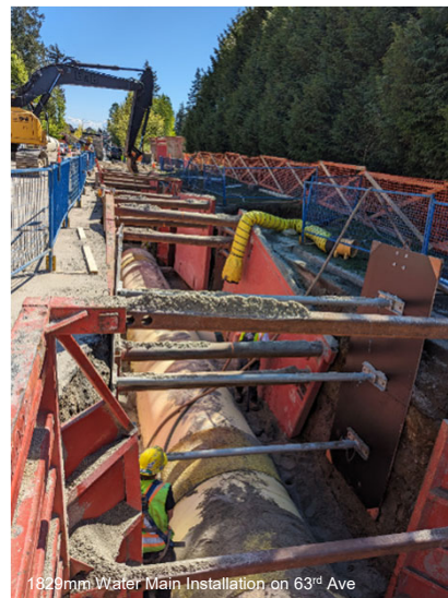
1829mm Water Main Installation on 63 rd Ave
