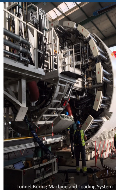
Tunnel Boring Machine and Loading System
