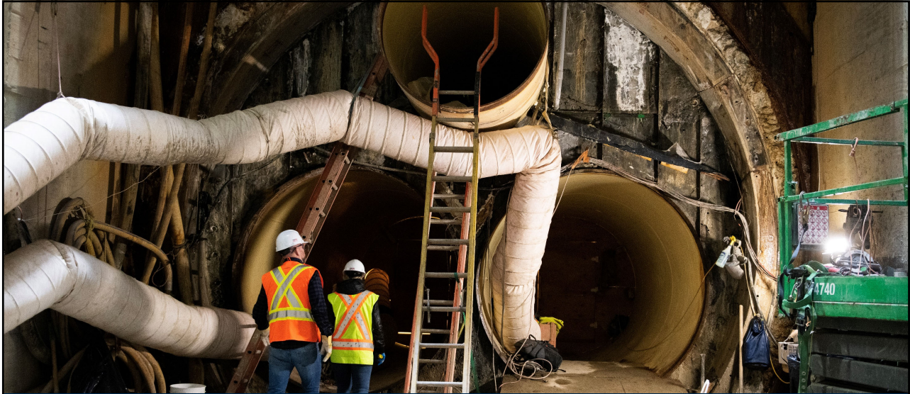
Workers inside the Second Narrows Water Supply Tunnel
