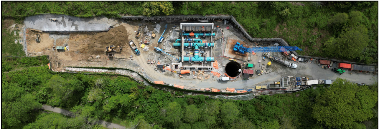
Overhead view of Second Narrows Water Supply Tunnel shaft
