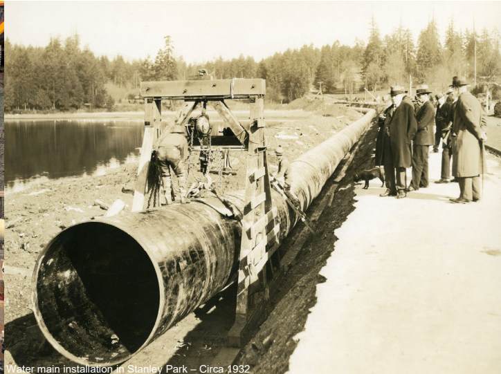
Water main installation in Stanley Park – Circa 1932
