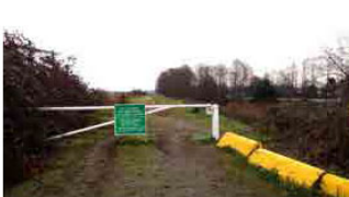
B. 152 ST SERVICE ROW NEAR MAIN ENTRY
