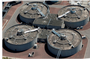
Annacis WWTP Digesters
