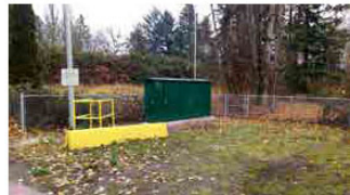
G. VIEW NORTH FROM INSIDE SIDE THE SITE
