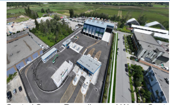
Central Surrey Recycling and Waste Centre
