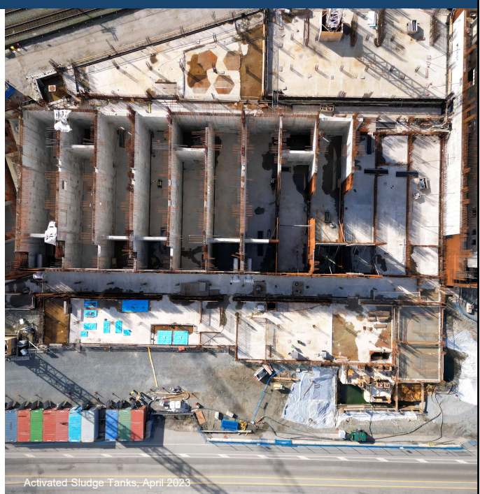
Activated Sludge Tanks, April 2023
