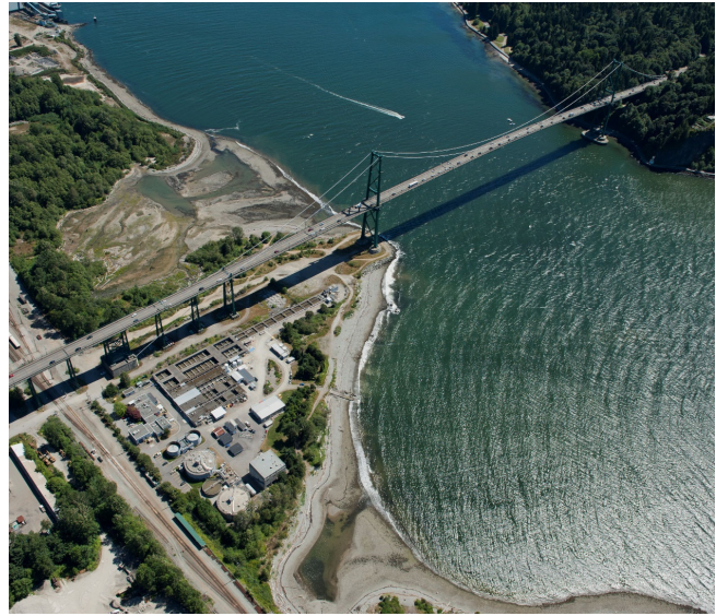
Lions Gate WWTP and Lions Gate Bridge, 2013
