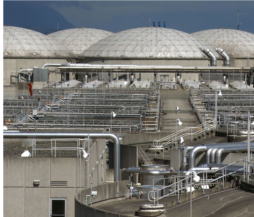
Annacis Island Wastewater Treatment Plant Trickling Filters
