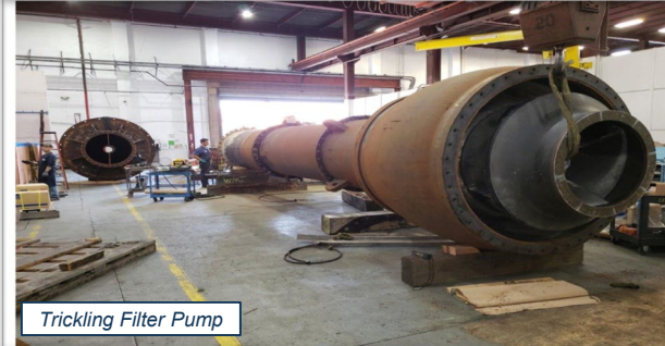
Sapperton Pump Station
