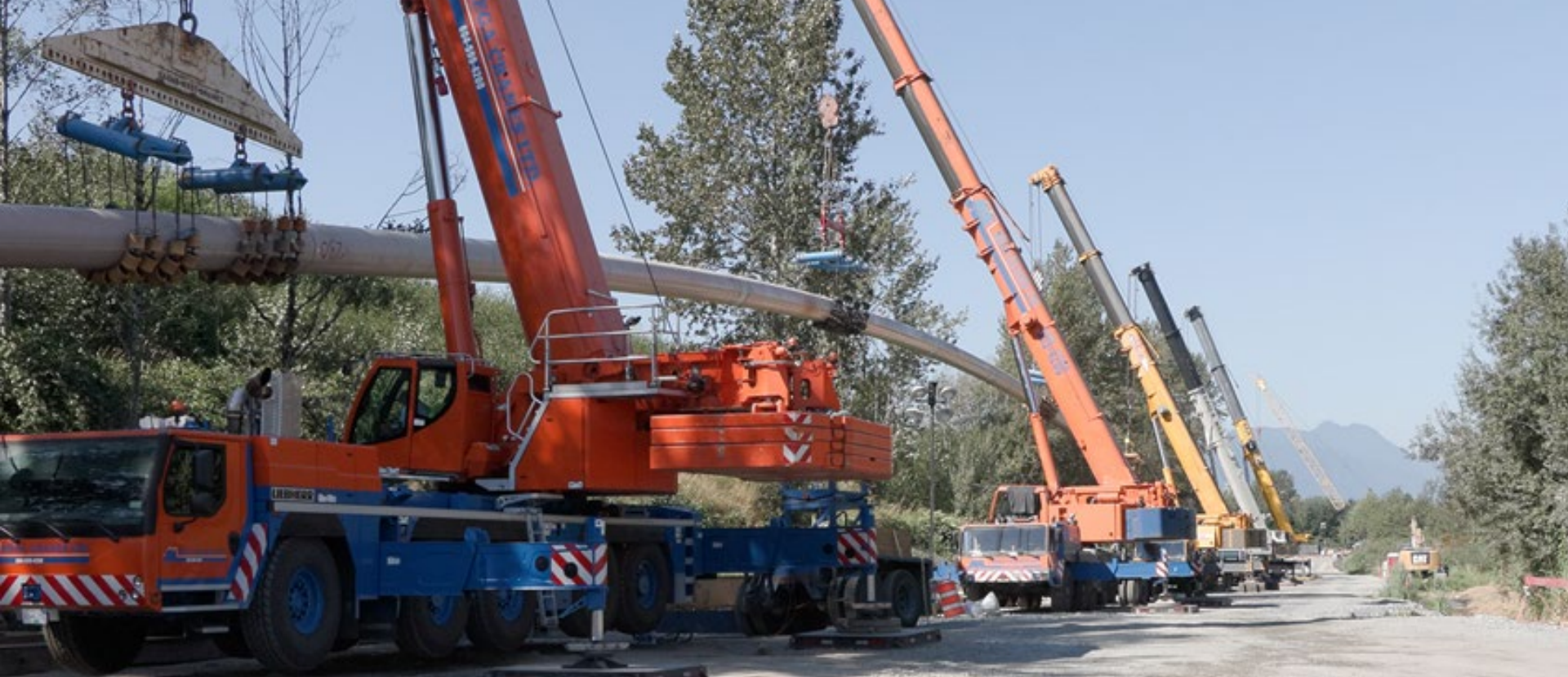
Fraser River Crossing pipe installation – Northwest Langley WWTP Projects
