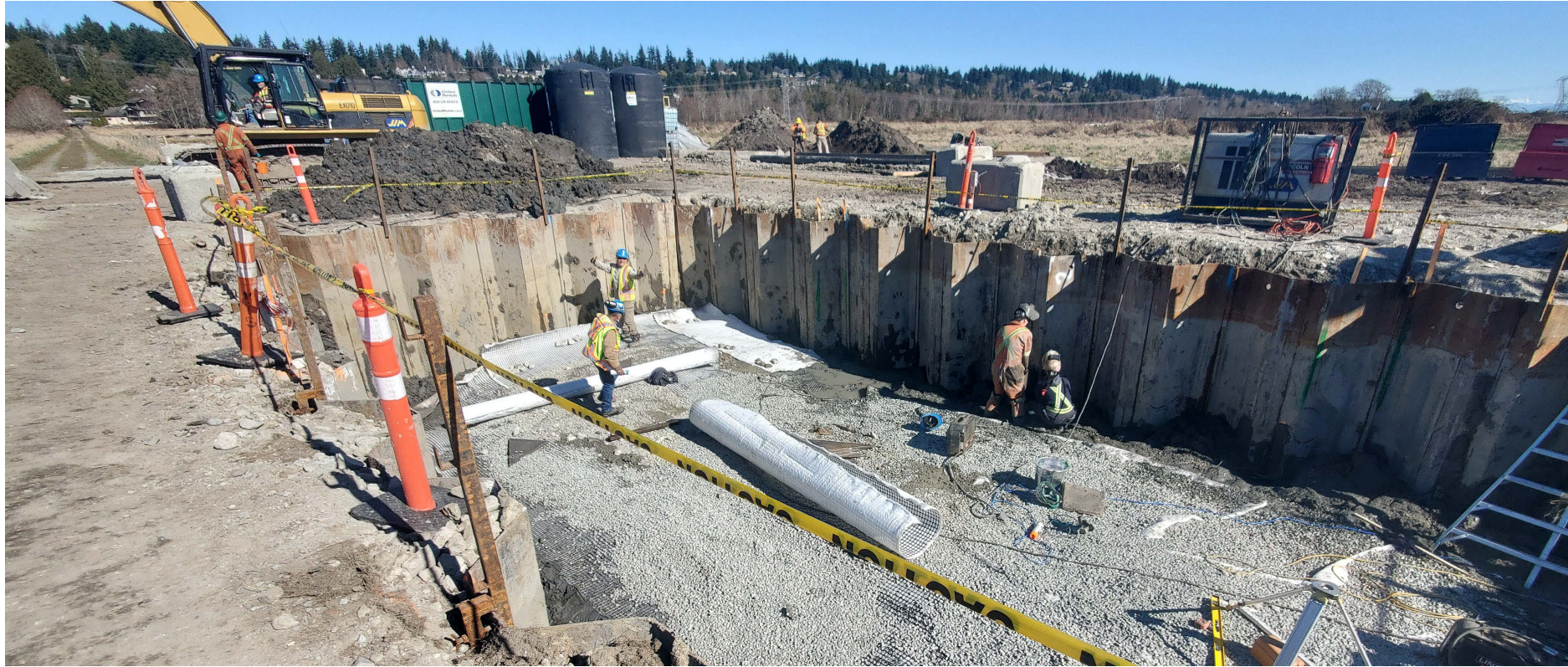
Crescent Beach Forcemain – Trenchless Section Launch Shaft
