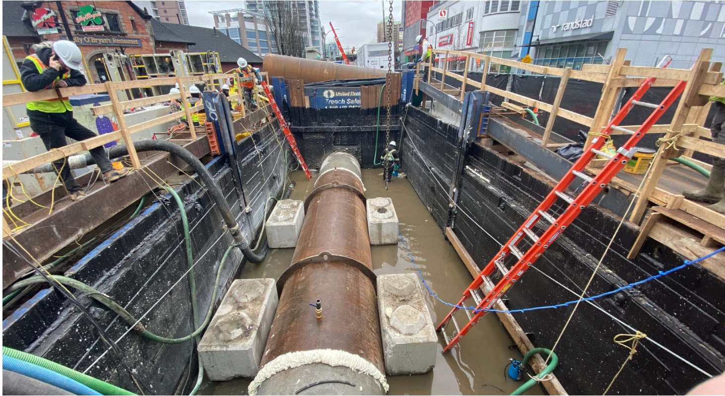
Pipe launch shaft at Columbia Street and 8 th Avenue
