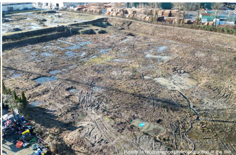
Ready to recommence pre-construction at the site
