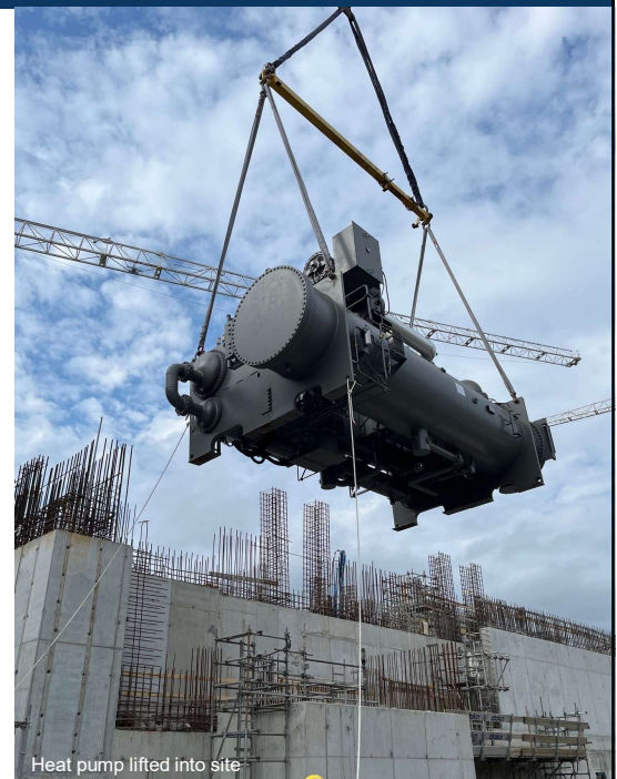
Heat pump lifted into site
