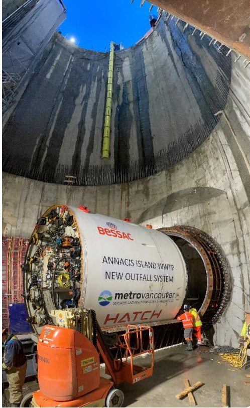
Figure 5: Launching the Tunnel Boring Machine (TBM)
