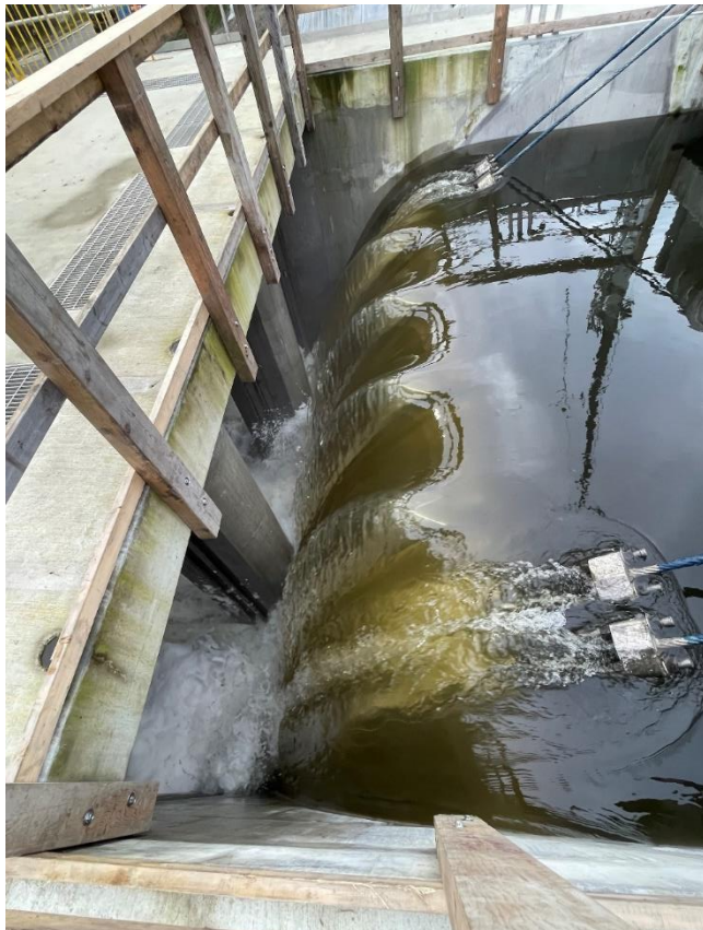
Figure 7: Treated Effluent flowing over the new control gate and into the new outfall system
