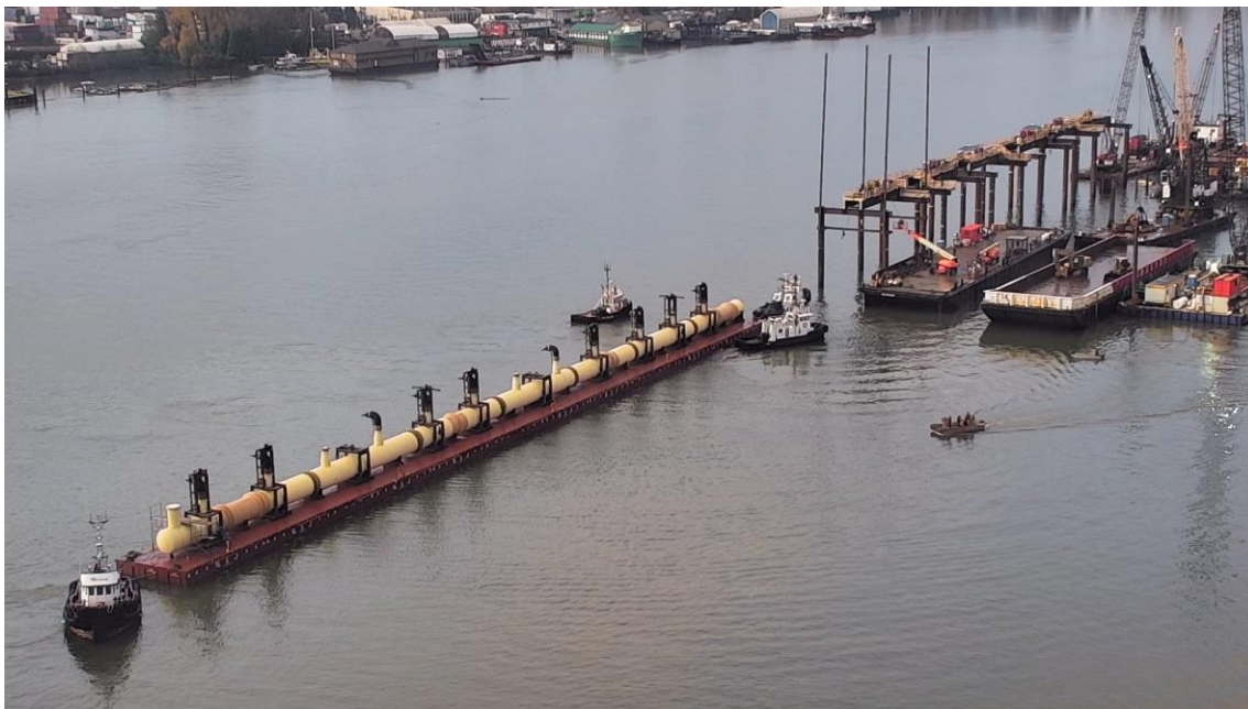
Figure 2: Positioning the east diffuser manifold before lowering it into a trench in the riverbed
