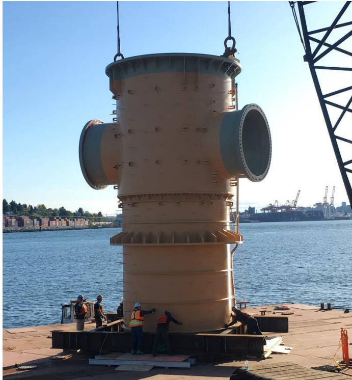
Figure 3: Placing the River Riser (it connects the deep tunnel to the diffuser manifolds)
