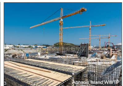
Annapolis Island WWTP
