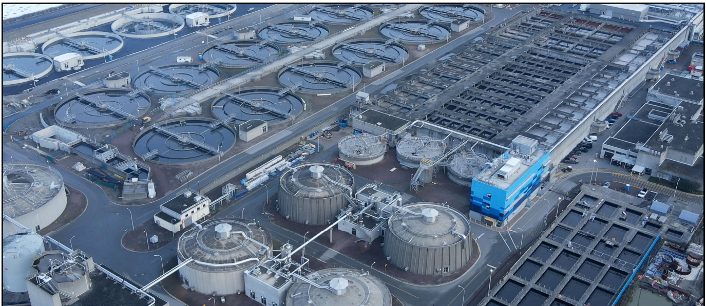
Annacis Island Wastewater Treatment Plant
