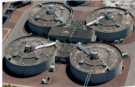
Annacis WWTP Digesters
