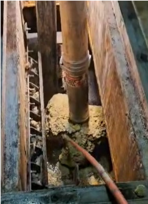
Grease Removal - Gilbert Trunk Sewer
