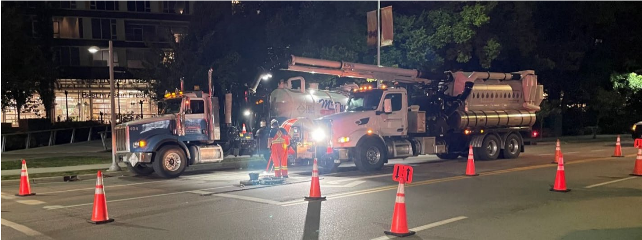
LWS Night-time Grease-removal Operation – Gilbert Trunk Sewer
