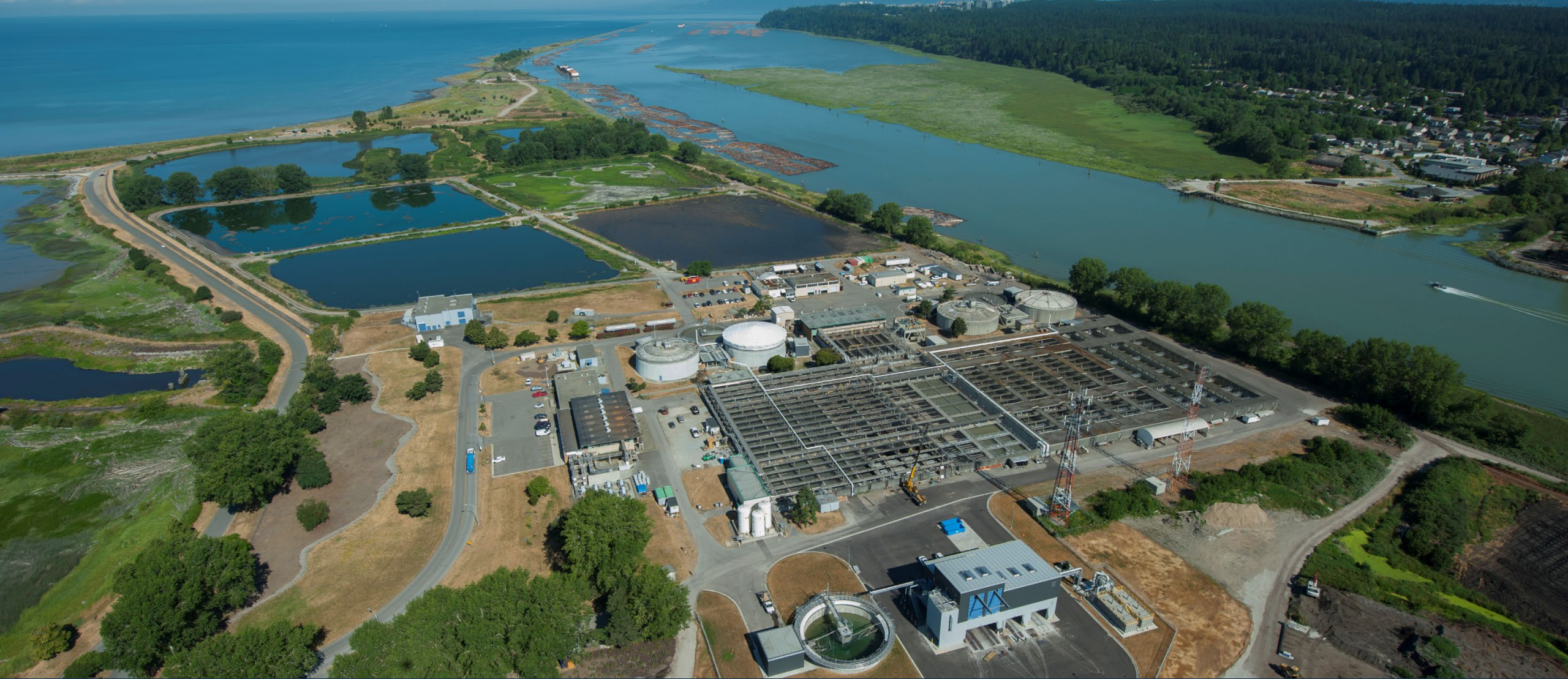
Iona Island Wastewater Treatment Plant
