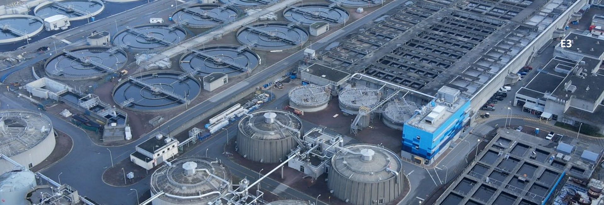
Annacis Island Wastewater Treatment Plant
