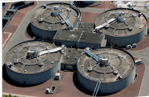
Annacis WWTP Digesters
