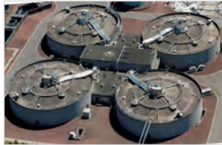
Annacis WWTP Digesters
