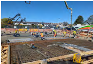
Fleetwood Reservoir Roof slab
