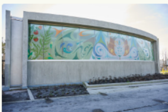
A glass mural at the new Metro Vancouver Fleetwood Reservoir, designed by Elinor Atkins
