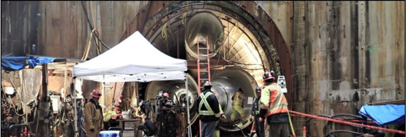
Second Narrows Water Supply Tunnel
