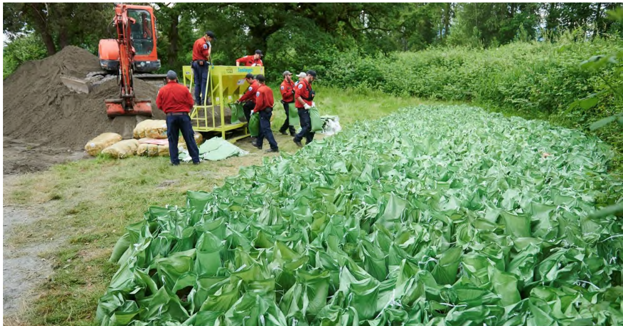
Figure 19: Watershed Protection staff filling a sea of sandbags on Barnston Island (Photo: Watershed Protection)
