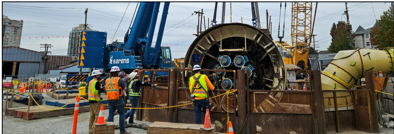
Annacis Water Supply Tunnel Boring Machine
