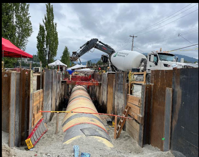
Coquitlam Water Main – Robson to Guildford Section
