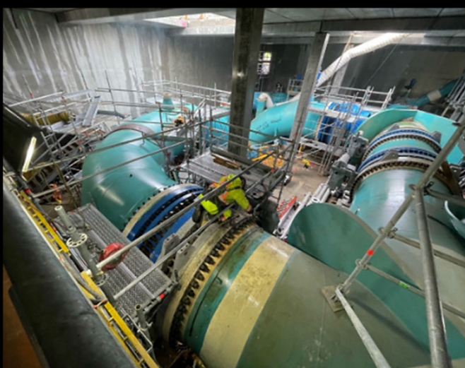
Second Narrows Water Supply Tunnel – North Valve Chamber
