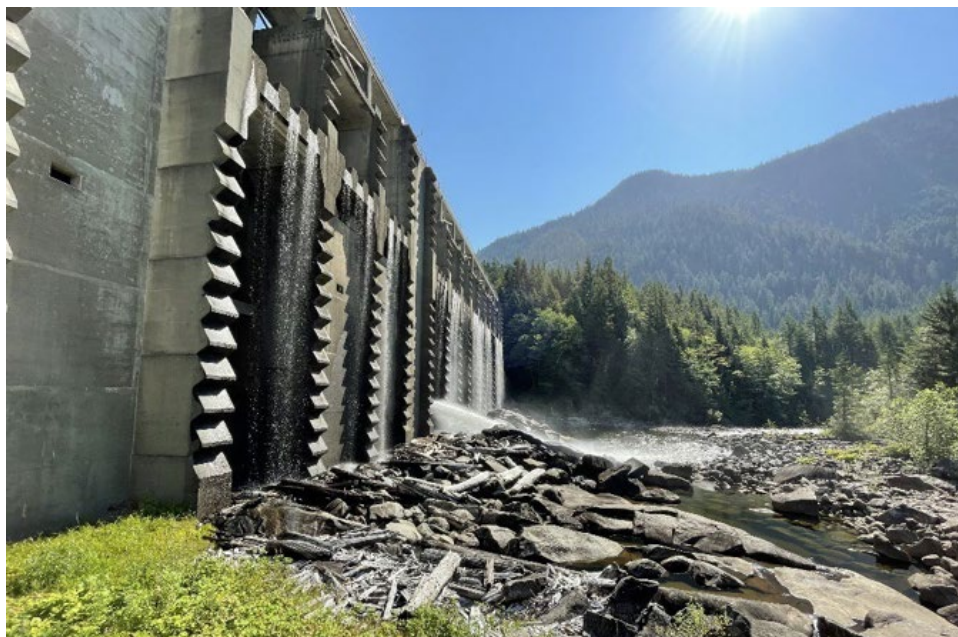
Seymour Falls Dam
