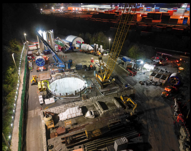
Annacis Water Supply Tunnel South Shaft
