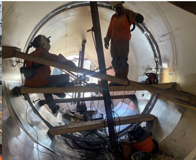
Robson to Guildford Section – 3.2m diameter steel pipe interior welding
