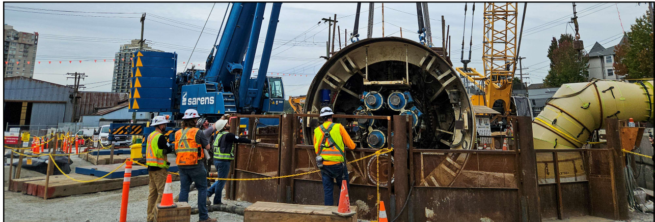
Annacis Water Supply Tunnel Boring Machine
