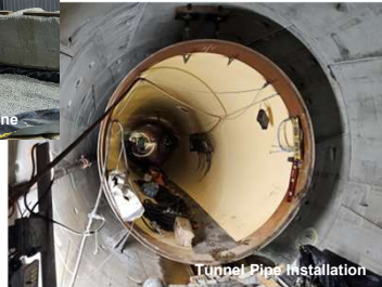
Tunnel Pipe Installation
