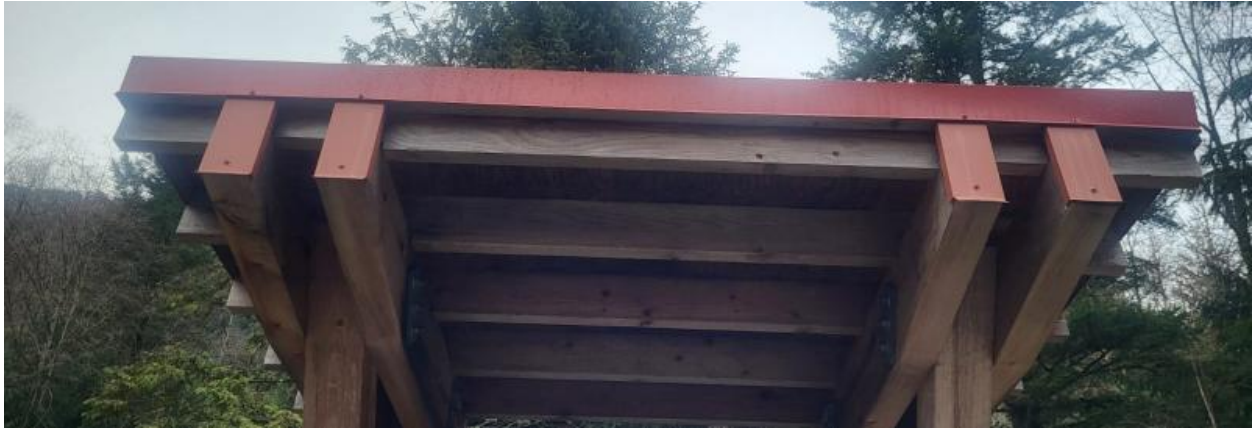
FIGURE 23 ROOF FLASHINGS FOR THE INFORMATION SIGNAGE
