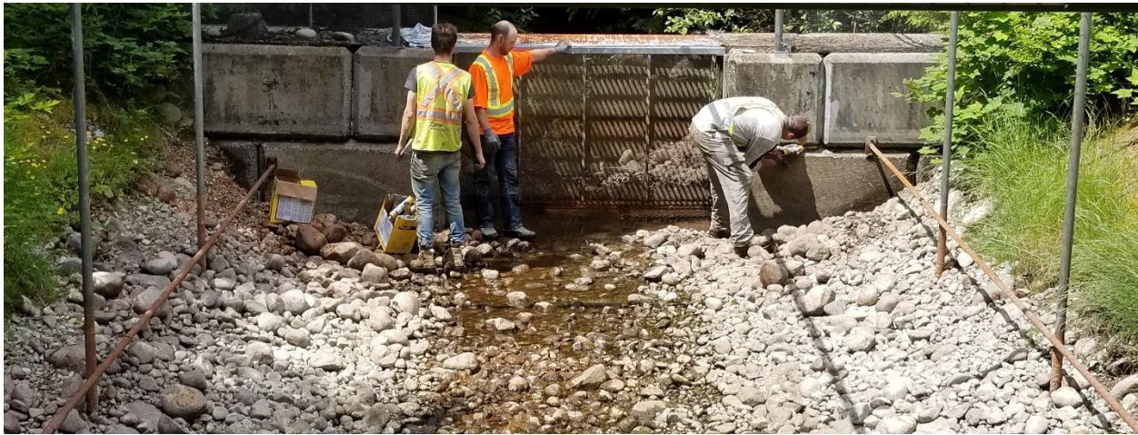
FIGURE 19 CONTRACTORS UNDERTAKING WEIR AND HEADWALL REPAIRS
