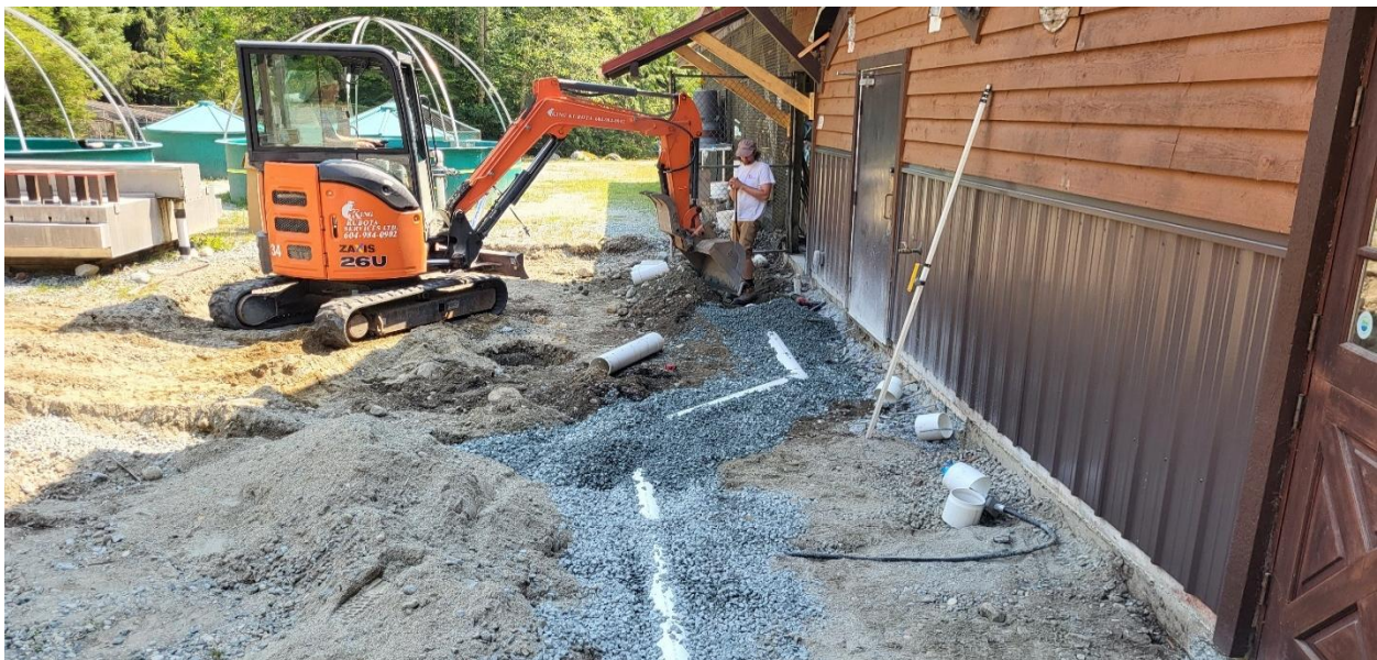
FIGURE 21 PERIMETER DRAINAGE WORKS AROUND HATCHERY BUILDING
