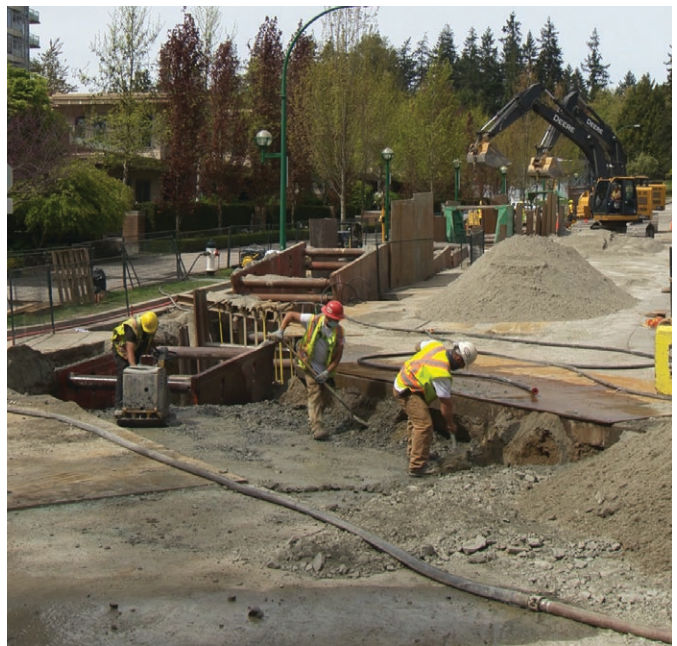
Central Park Water Main construction
