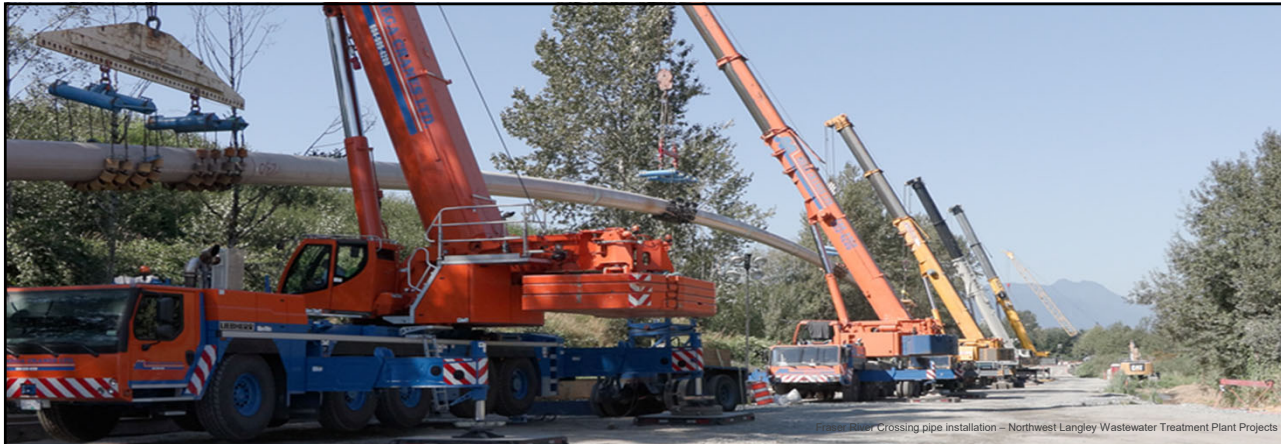
Fraser River Crossing pipe installation – Northwest Langley Wastewater Treatment Plant Projects
