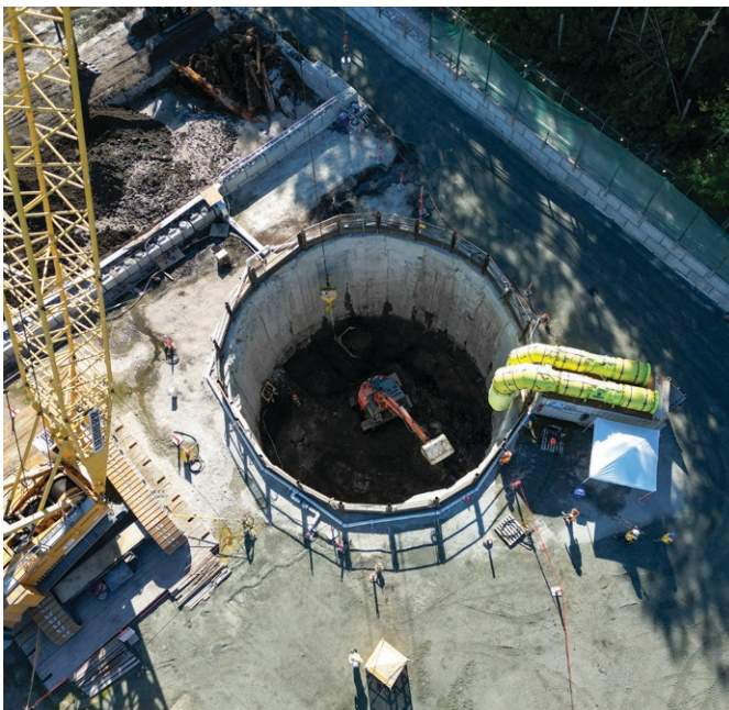
Annacis Water Supply Tunnel construction
