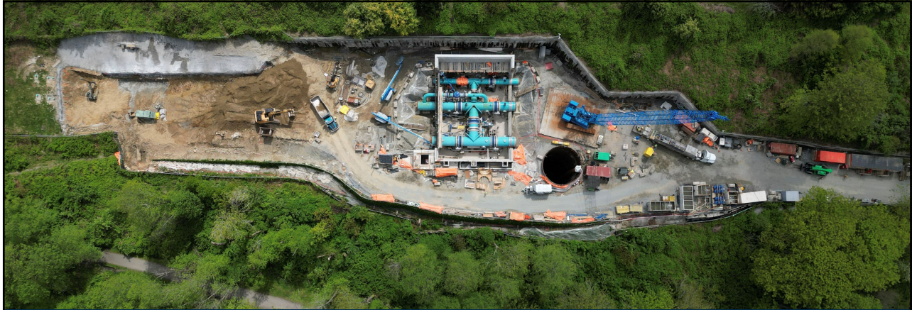
Overhead view of Second Narrows Water Supply Tunnel shaft
