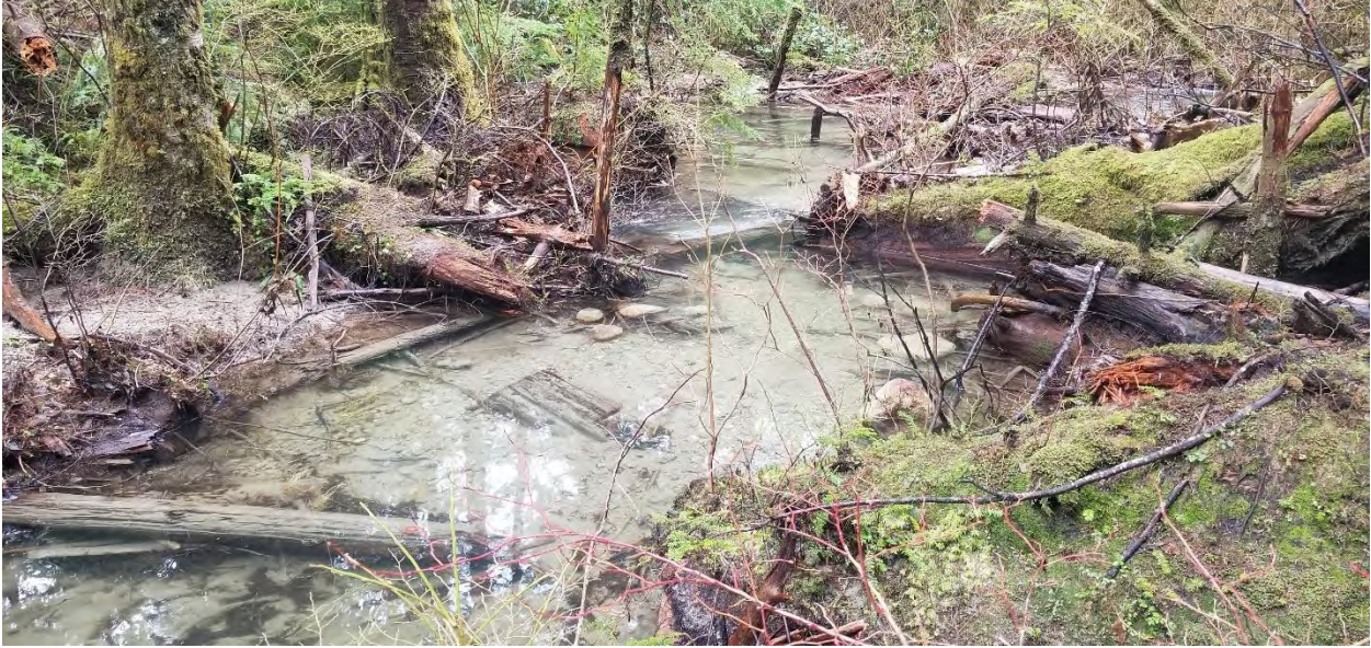
FIGURE 2 JUNIOR CREEK FOLLOWING COMPLETION OF REPAIR WORKS VIEWED DOWNSTREAM
