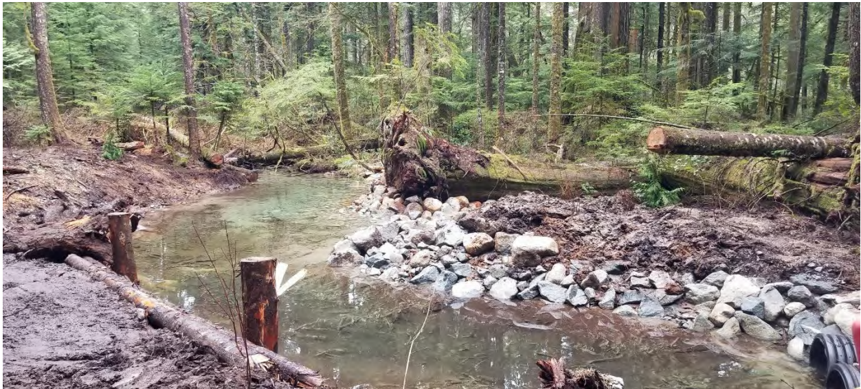
FIGURE 1 JUNIOR CREEK FOLLOWING COMPLETION OF REPAIR WORKS VIEWED UPSTREAM
