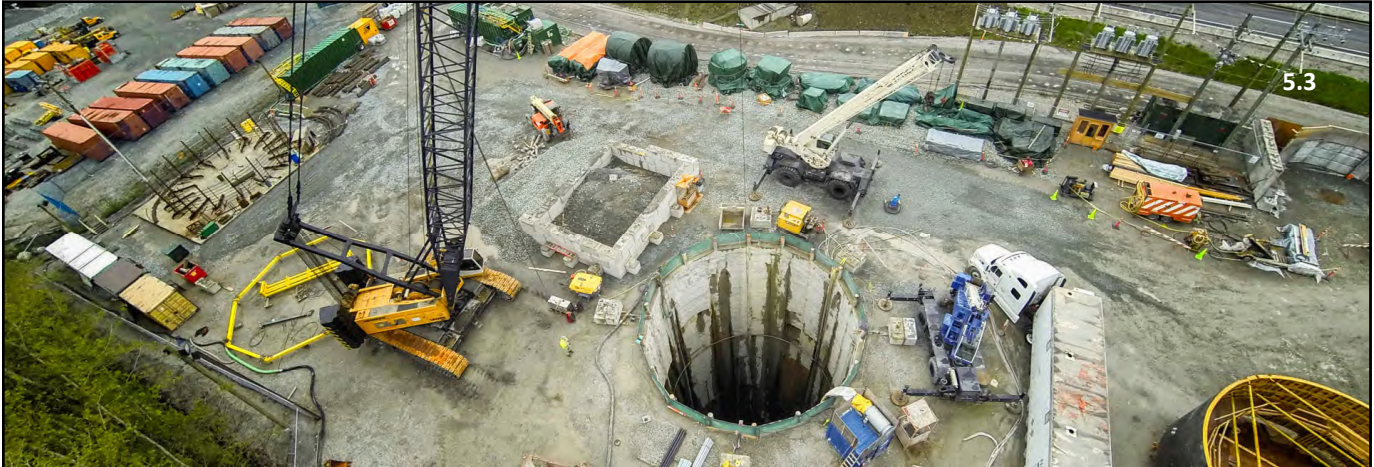
Port Mann Water Supply Tunnel Shaft
