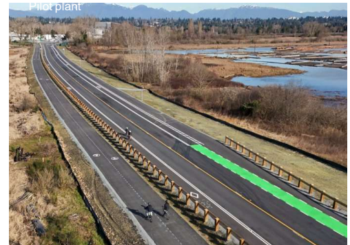
Causeway improvements completed
