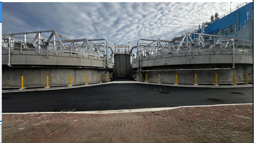
New Gravity Thickeners 4 and 5
