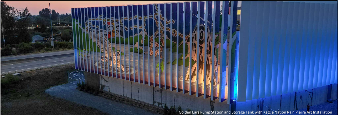
Golden Ears Pump Station and Storage Tank with Katzie Nation Rain Pierre Art Installation
