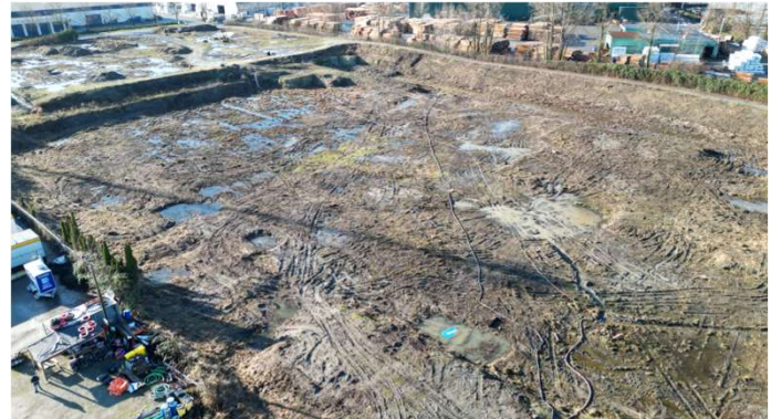
WWTP site – ready to recommence pre-construction
