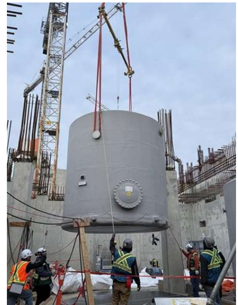
Chemical storage tank installation
