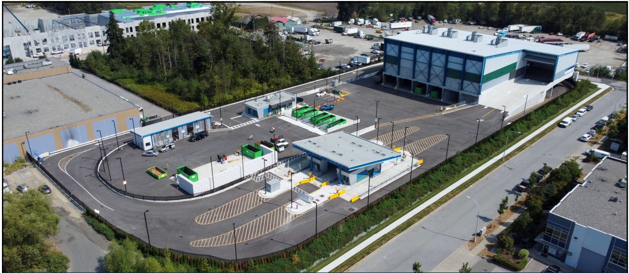
Central Surrey Recycling and Waste Centre
