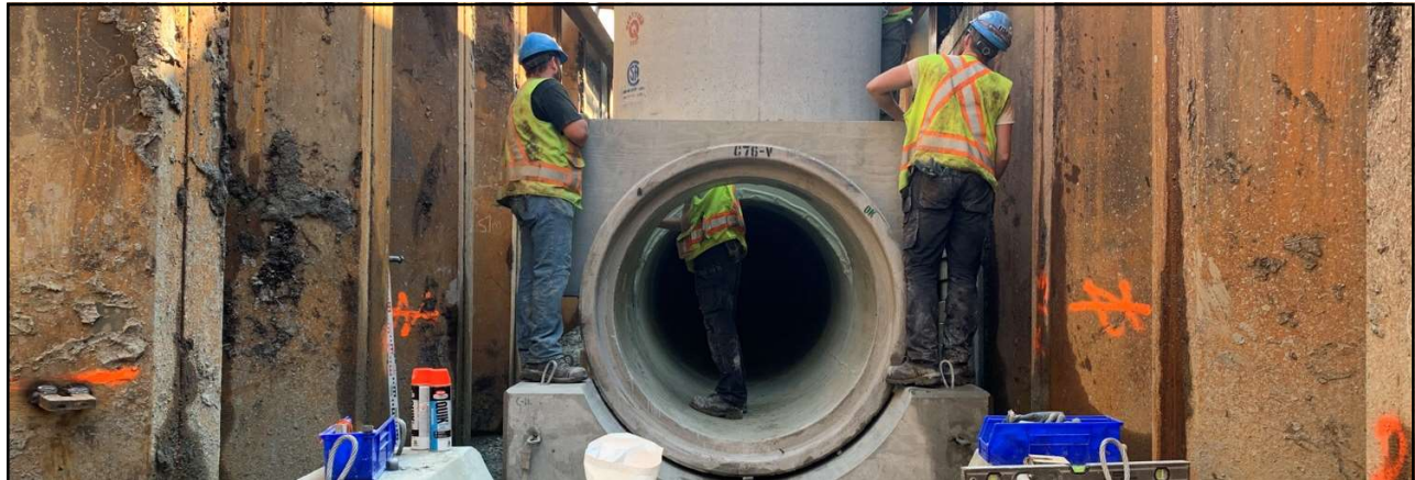
Winston Street Sewer Construction
