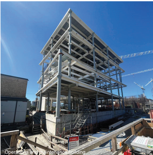
Operations and maintenance building
