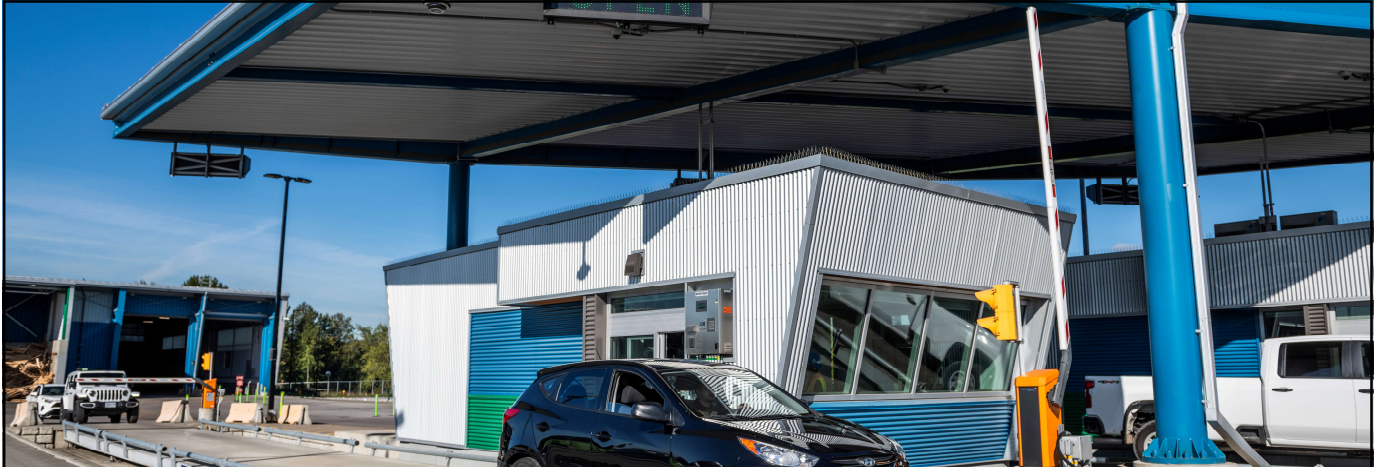
United Boulevard Recycling and Waste Centre
