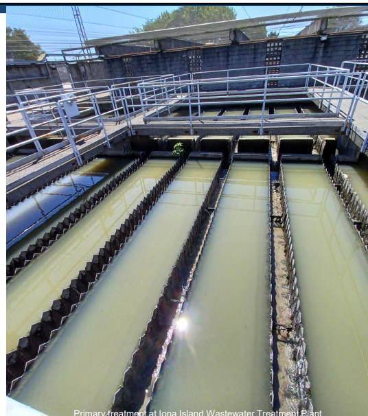
Primary treatment at Iona Island Wastewater Treatment Plant
