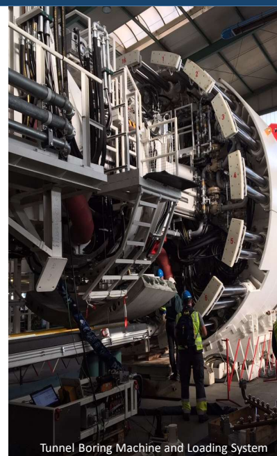
Tunnel Boring Machine and Loading System
