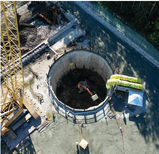
Annacis Water Supply Tunnel construction
