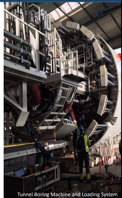
Tunnel Boring Machine and Loading System
