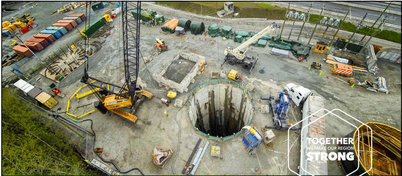
Port Mann Water Supply Tunnel
