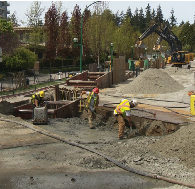
Central Park Water Main construction
