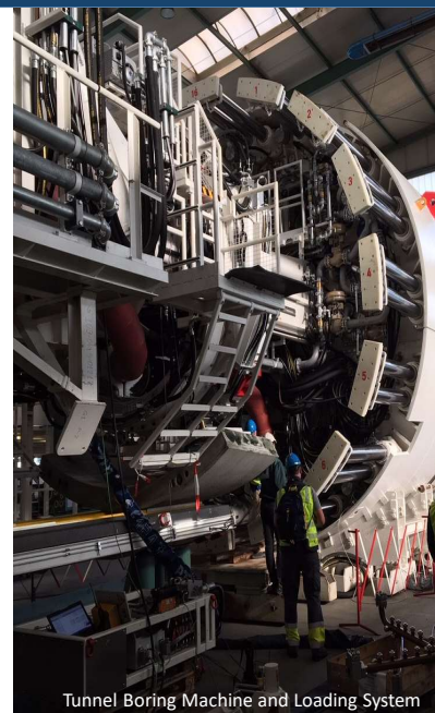
Tunnel Boring Machine and Loading System
