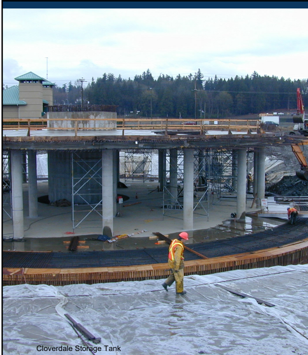
Cloverdale Storage Tank
