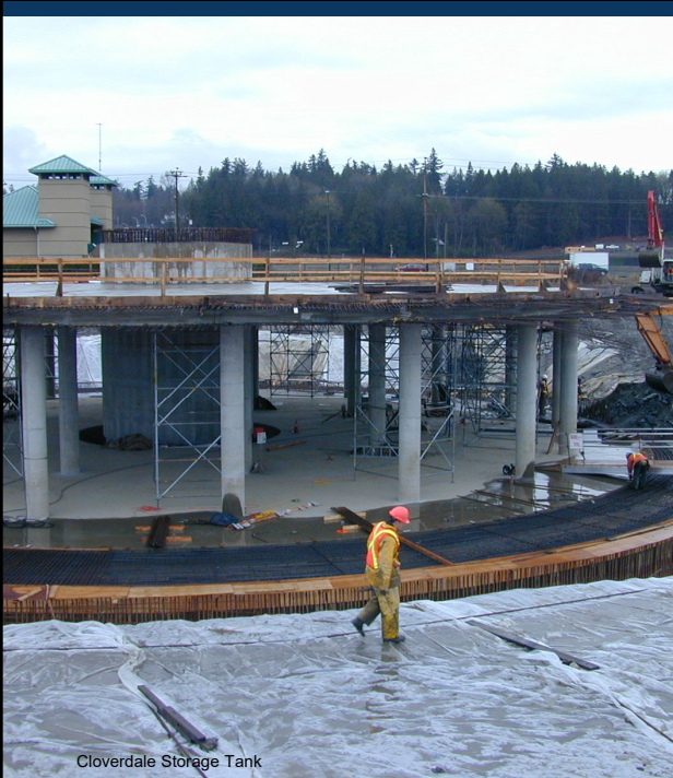
Cloverdale Storage Tank
